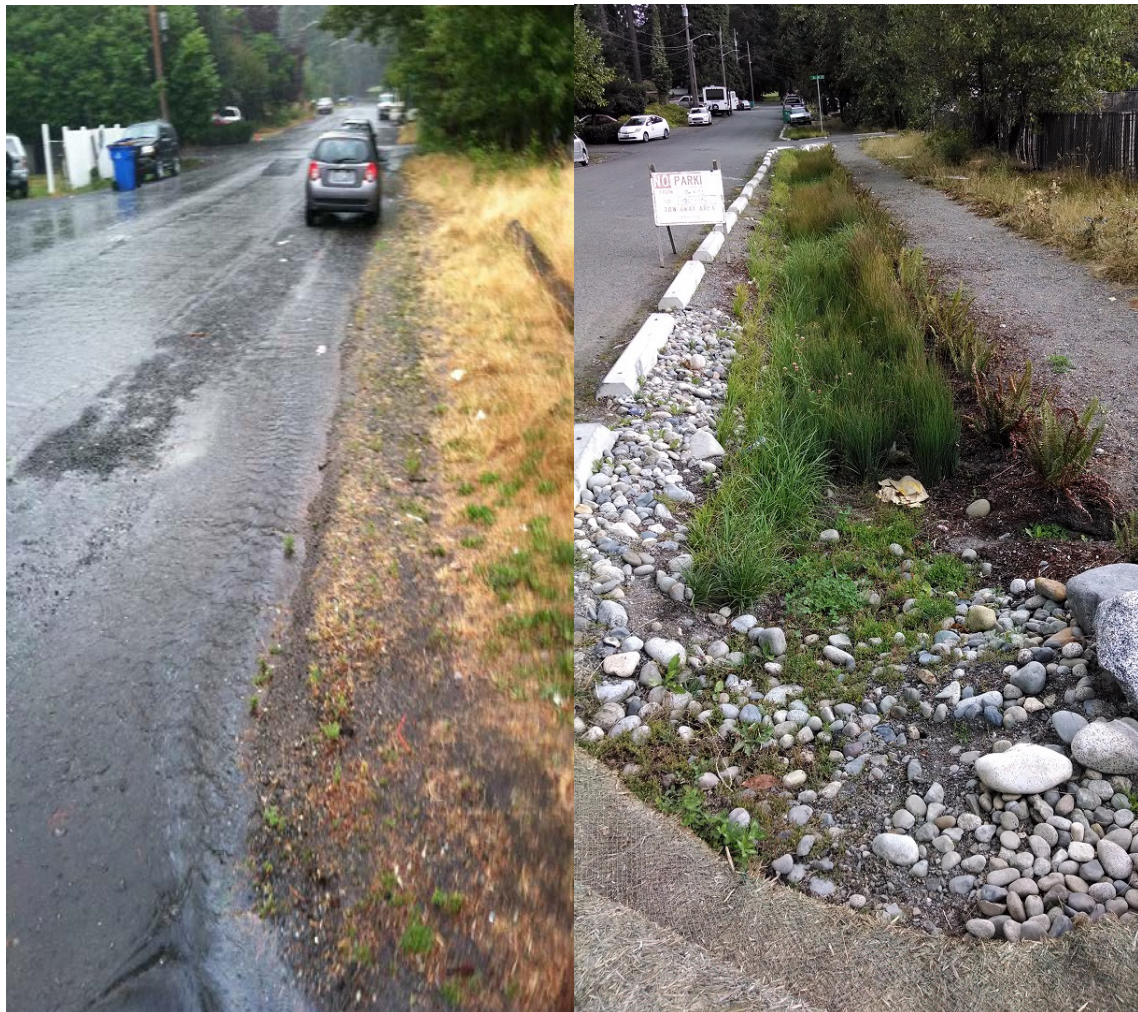
Figure 1. 32 nd Ave NE and NE 147 th St Greenworks Bioretention Project, Before and After
