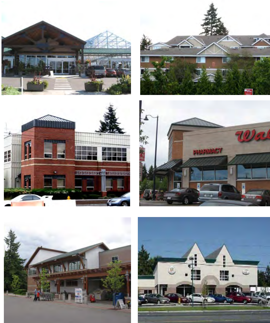
Fig. 16 A variety of existing roof shapes, materials, and colors in Town Center
