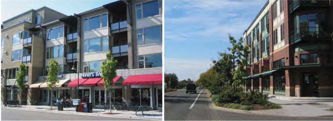
Storefront and Boulevard buildings
