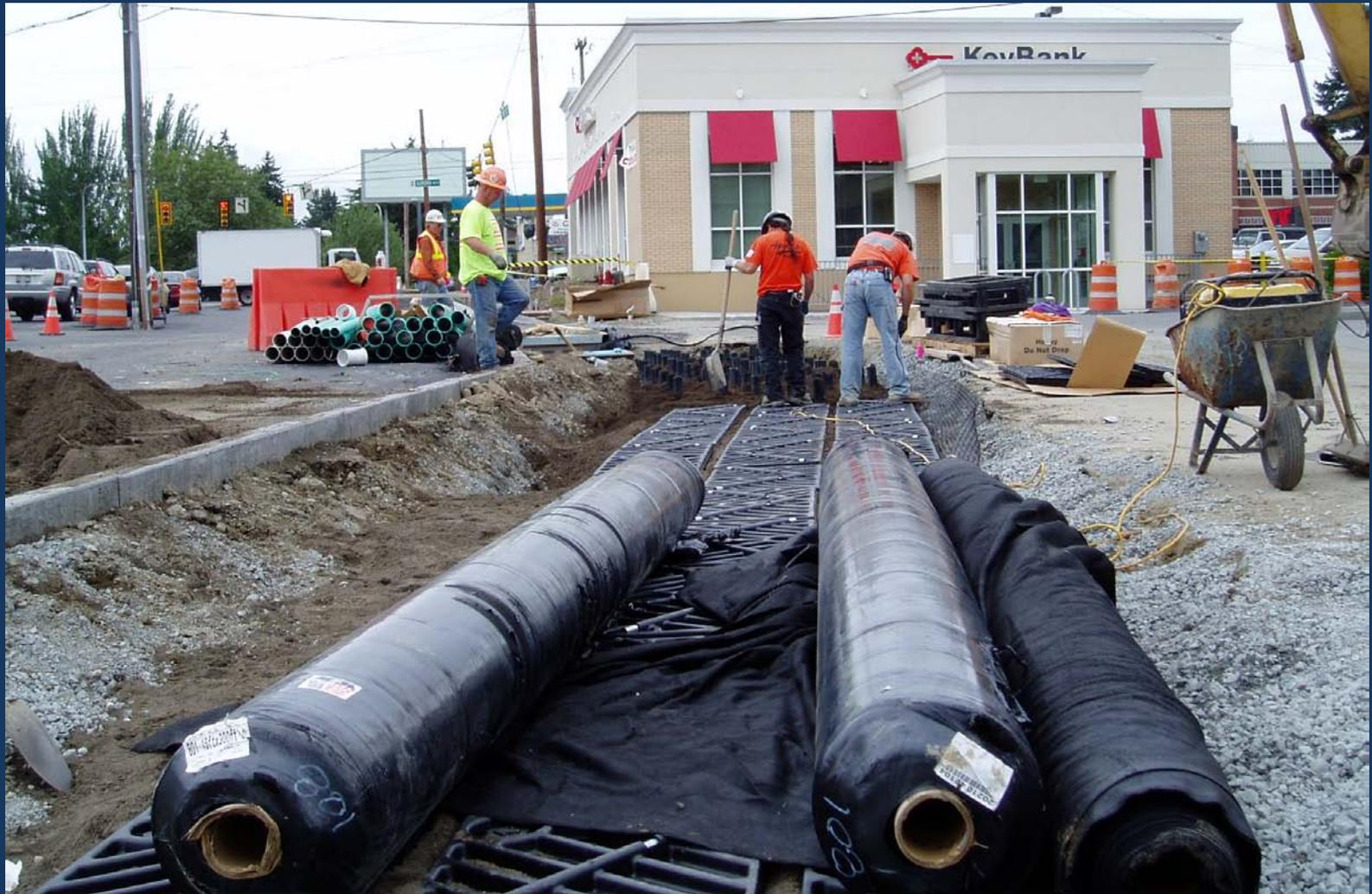
Geotextile material is placed over the entire system.
