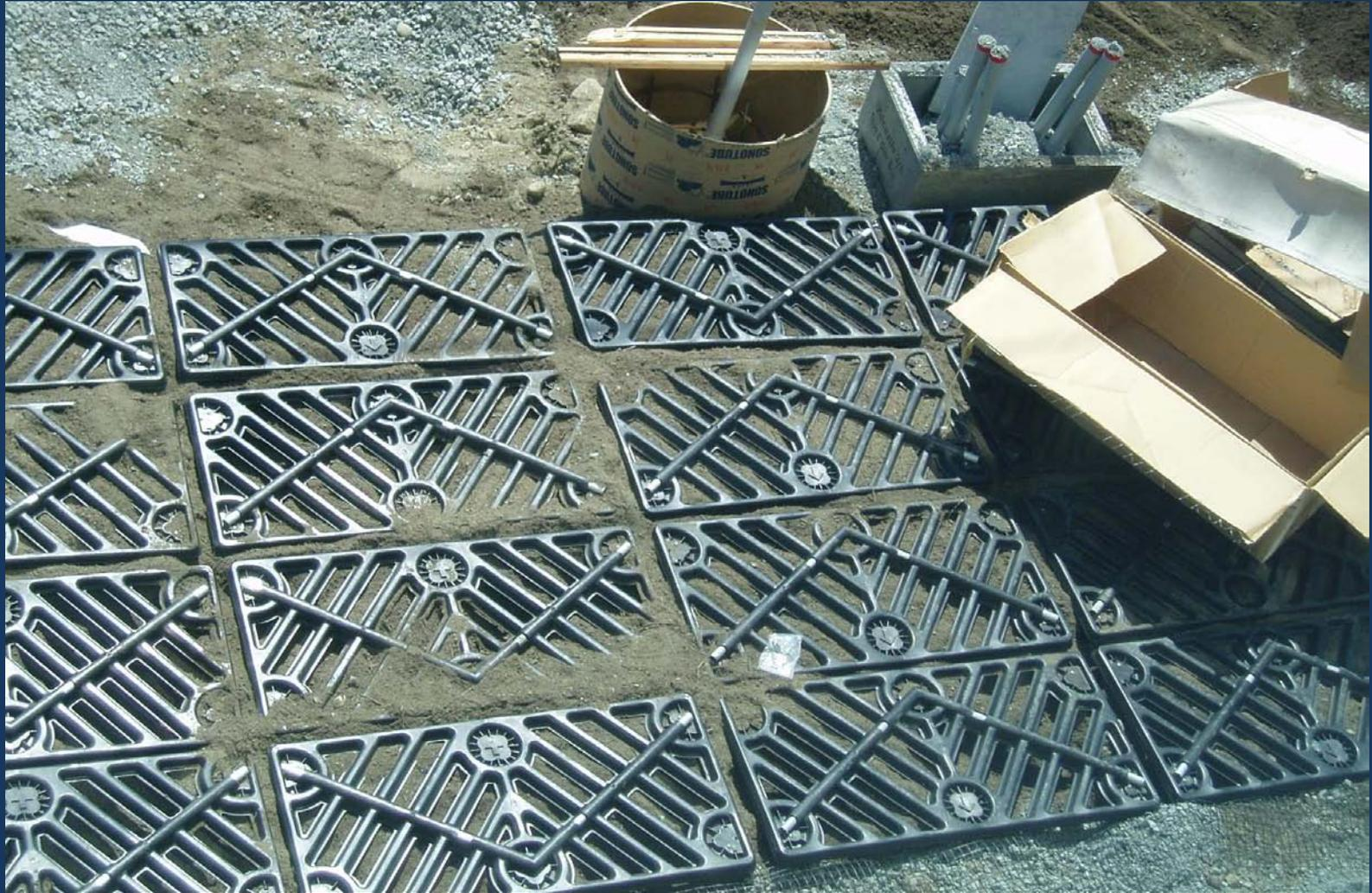
The deck is a rigid platform with ample openings for air and water penetration. Two diagonal channels house galvanized steel tubes to help prevent deformation.
