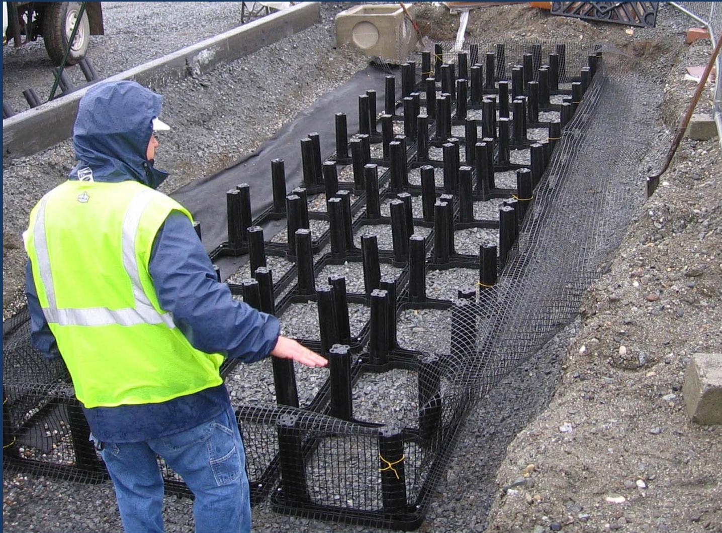
Geogrid is placed around the entire system to properly hold soil in place.
