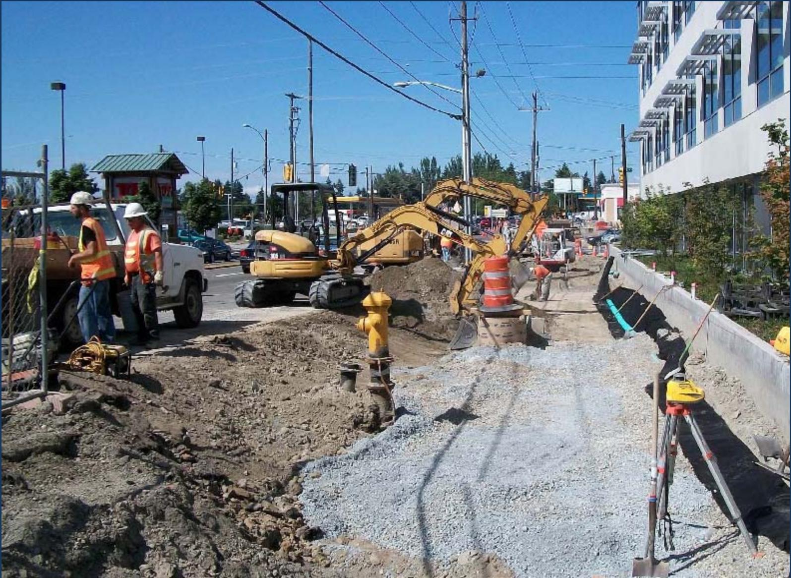
A sub base aggregate is placed in the excavated trench and compacted.
