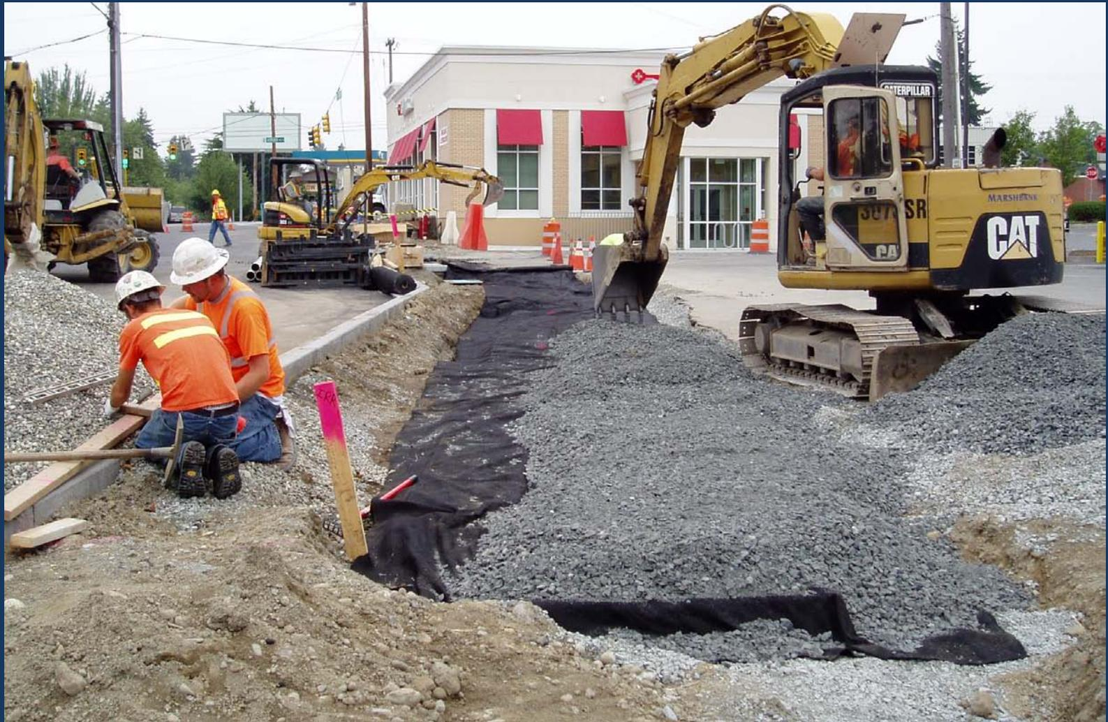
An aggregate base course is placed on top of system.
