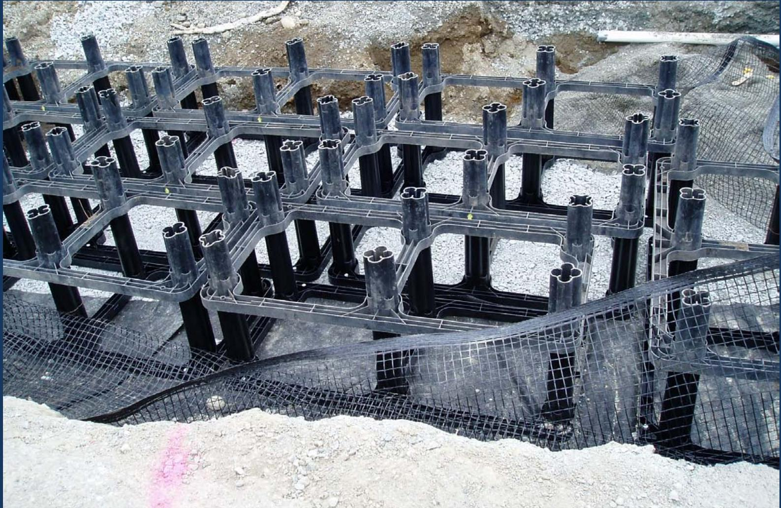
“Strongbacks” are placed on top of frames. They are only required during installation and compaction of soil to help hold frames in place .
