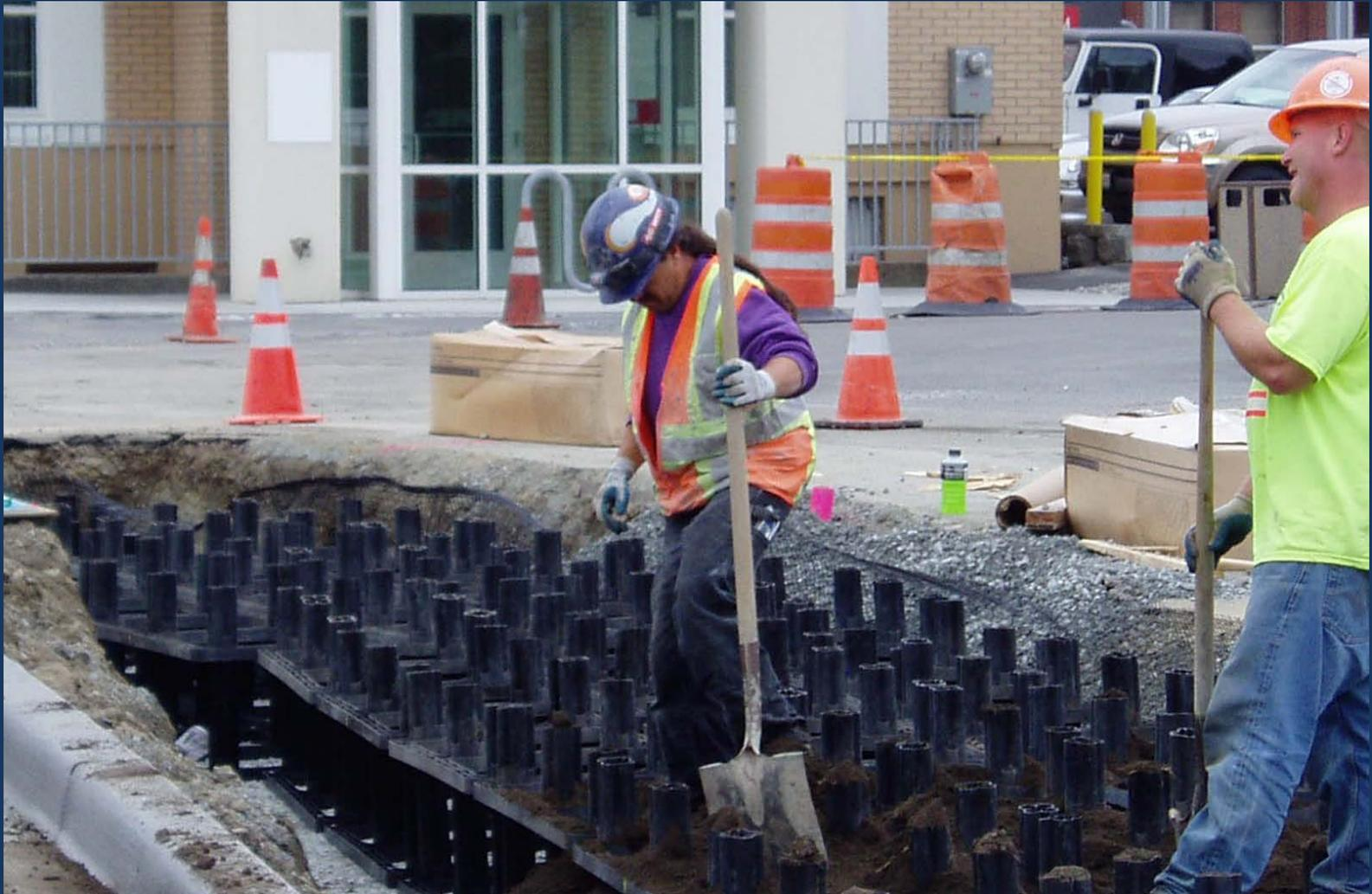
Soil is spread with shovels and compacted by foot.
