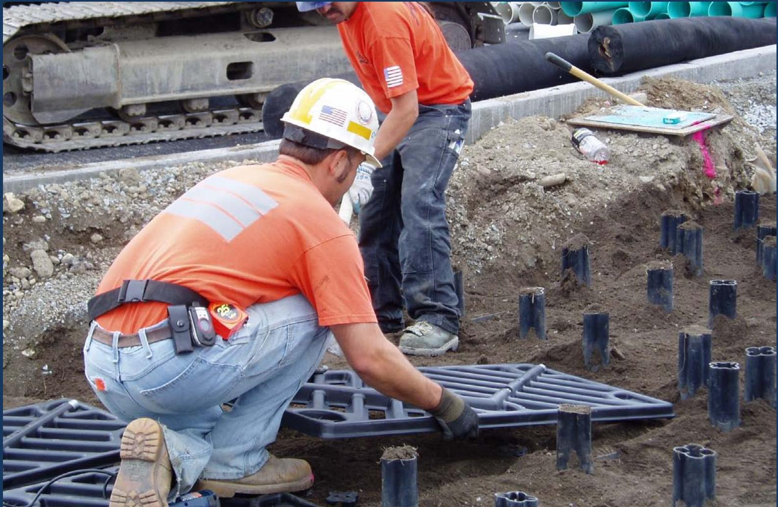
The deck is put into place right after the strongback is removed.
