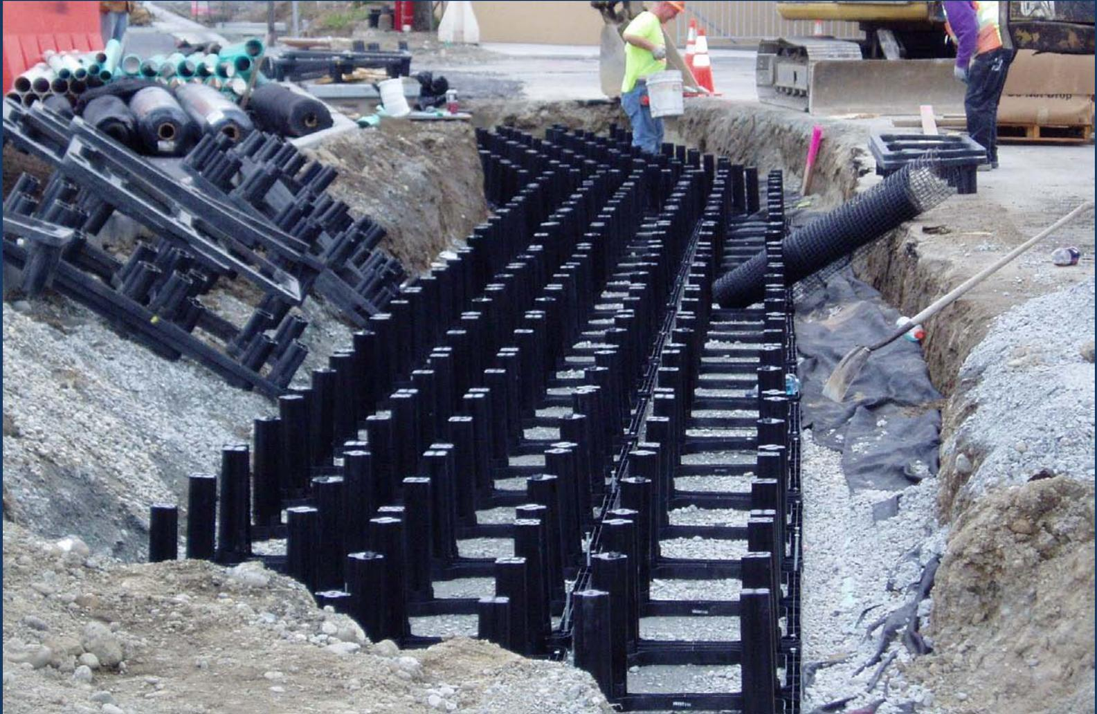
A network of frames (each with six rigid vertical posts) is positioned on the base material and anchored in place. These frames can be stacked one, two, or three high allowing for varying capacity.
