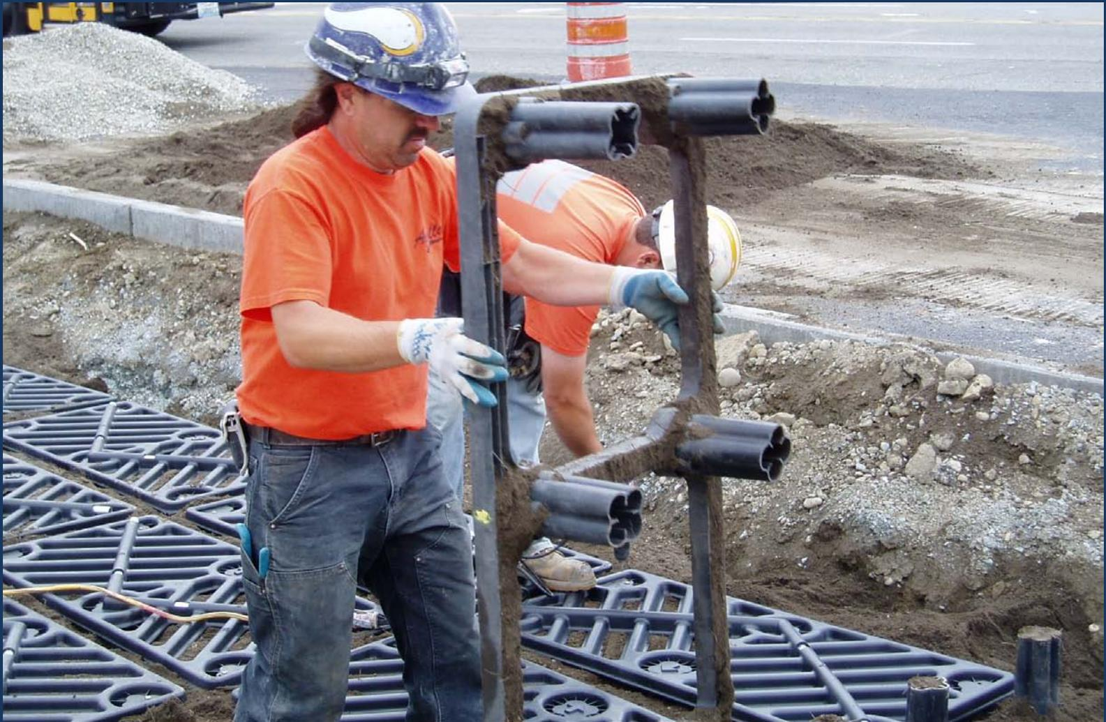
Strongbacks are moved and reused as the work progresses.
