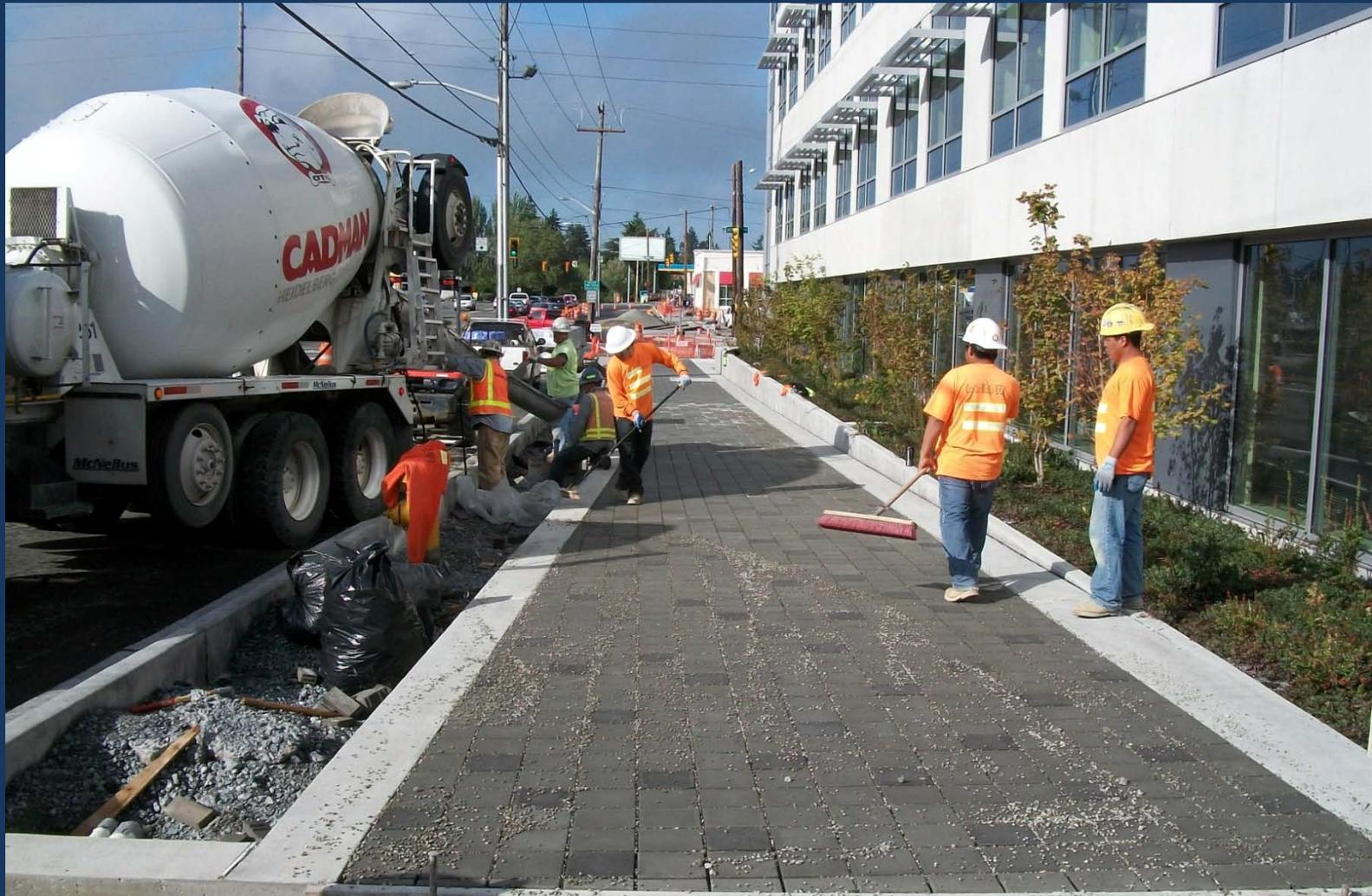
For this portion of the project, pavers spaced with gravel (allowing for infiltration) are placed over the newly installed root box system for a public sidewalk. Trees will be planted soon.
