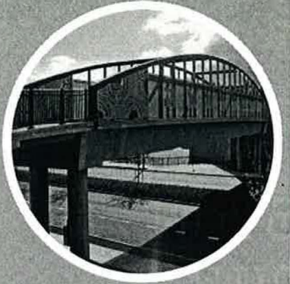
Aurora Pedestrian Bridge
