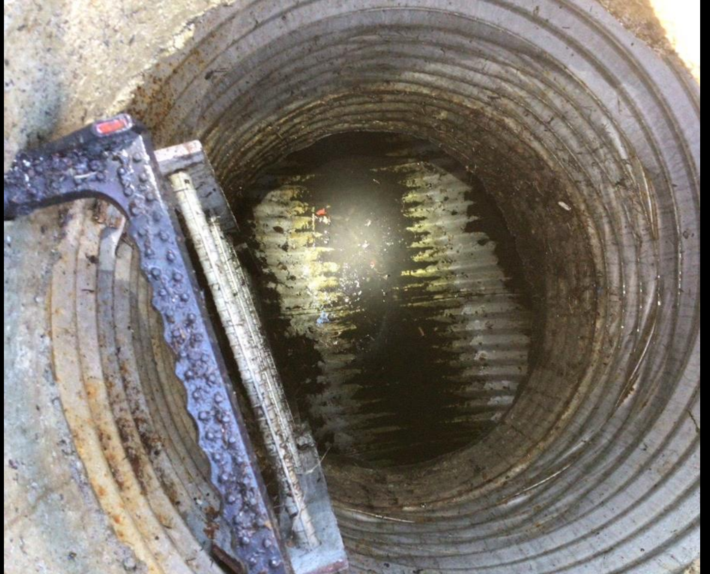
A detention pipe as viewed from ground level via access maintenance hole.
