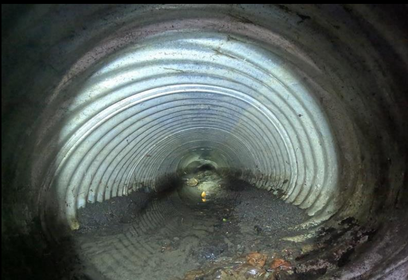
Above: Clean detention Pipe Below: Excessive sediment in pipe, needs maintenance.
