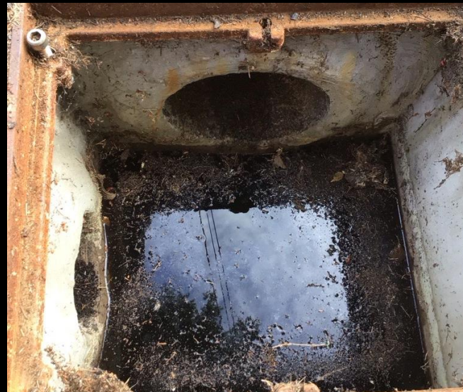
Interior Photo with 12" concrete pipes
