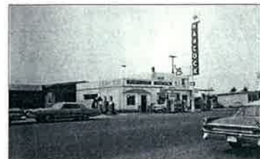
The original service station, now Texaco
