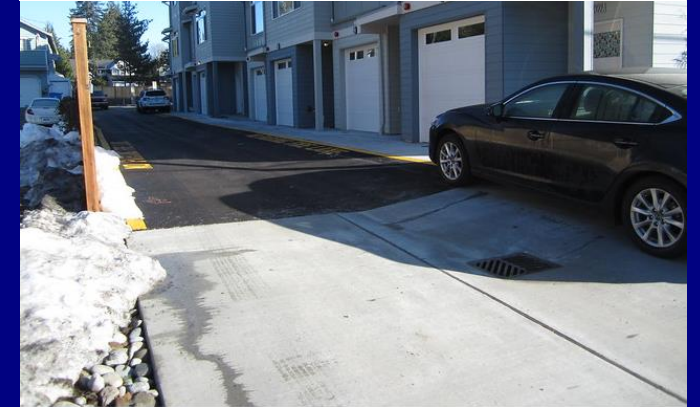
Ranked #3: Pedestrian access next to driveway
