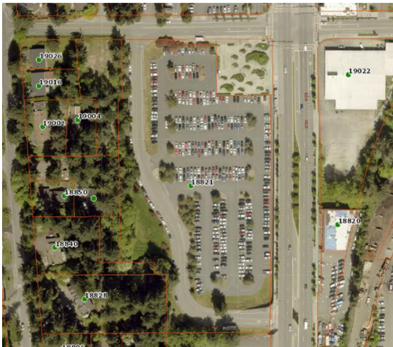
Figure 3 Park N Ride Existing Condition (2019 aerial photo)
