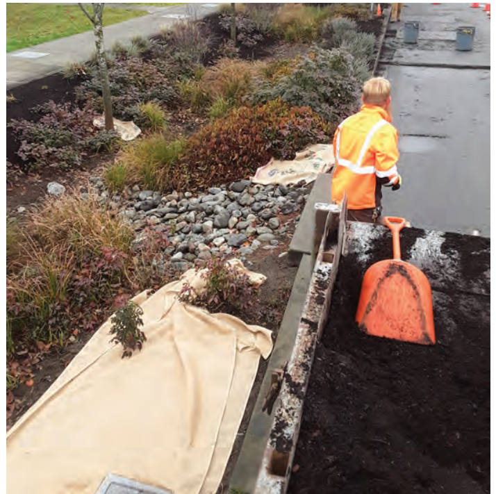
Grounds Maintenance workers applying compost and burlap to a bioretention bed along Aurora Avenue.
