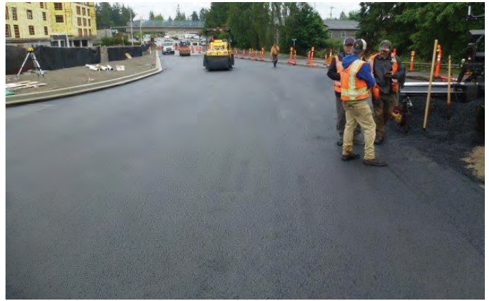
Paving the intersection of Westminster Way N and N 155th Street.
