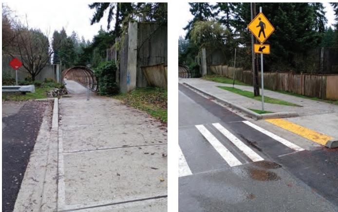
Left: The shared-use sidewalk to the pedestrian bridge over I-5. Right: The new crosswalk and curb ramp.
