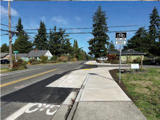
Top left: Before (top) and after (bottom) photos of the project at 1st Avenue NE and N 192nd Street.
