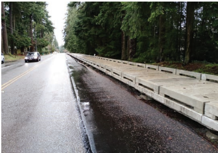
The completed elevated walking path at Dayton Avenue N.
