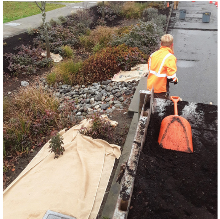
Grounds Maintenance workers applying compost and burlap to a bioretention bed along Aurora Avenue.
