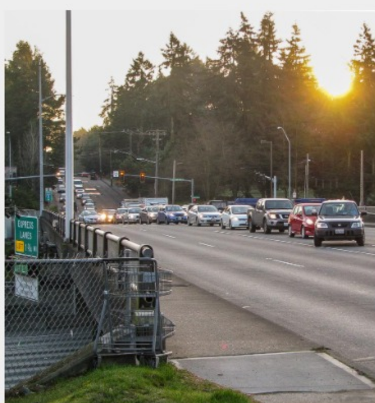
145th Street, looking west across the bridge over I-5
