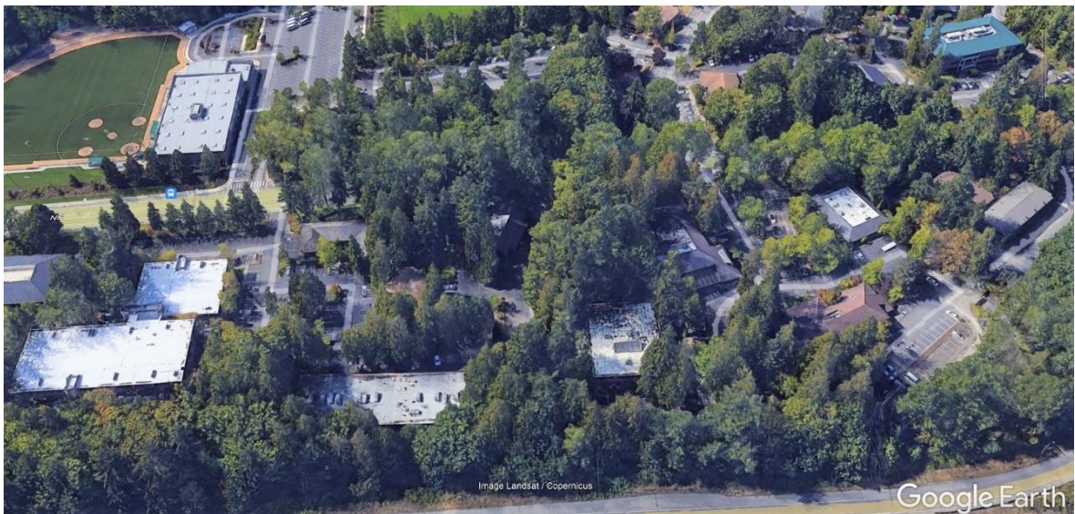
A commercial Office Park in Bellevue with thoughtfully-integrated mature Significant Trees (credit: Google Earth)
