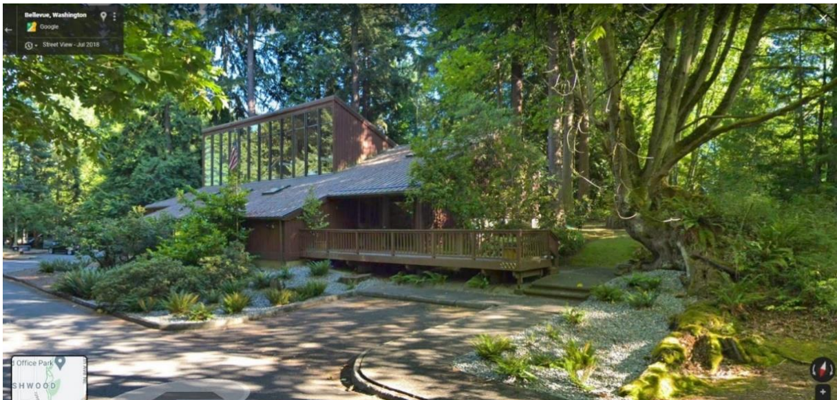
The integration of Significant Trees creates a symbiotic relationship between the Natural and Built Environment (credit: Google Street View)
