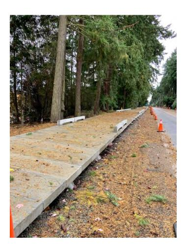
2. In 2009 Shoreline required this construction of the sidewalk adjacent to the new Southwoods Park on NE 150<sup>th</sup>. It included a section of pervious pavement and worked around existing trees and also included new plantings of native Dogwood Trees.
