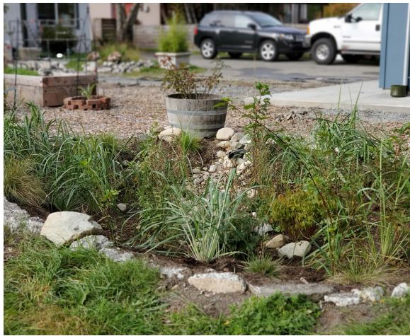
PHOTO: Rain garden in Ridgecrest neighborhood soaks up rain runoff from a roof, deck, and driveway, filtering pollutants from tire and roof particles, car leaks, and other types of pollution.
