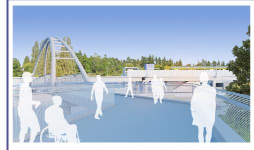
**TIED ARCH BRIDGE:** Stretching over I-5, the side-by-side arches and supporting cables of the bridge will create space and light for people using the bridge and those traveling nearby. The bridge will be wide enough for pedestrians and bicycles and built to comply with American with Disabilities Act (ADA) standards.
