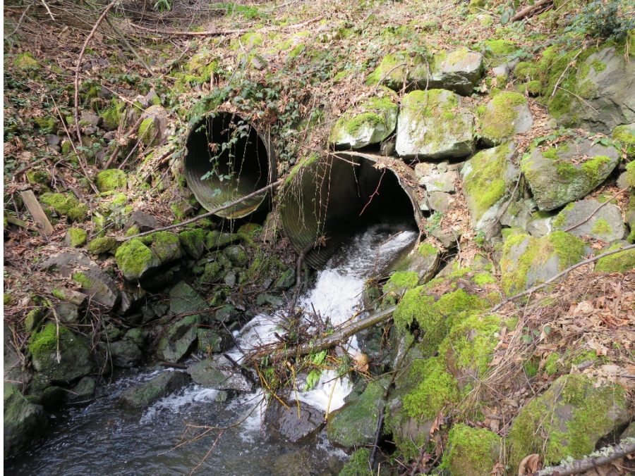
Figure 2. Outlet Conditions of Boeing Creek Culverts Beneath NW Innis Arden Way.
