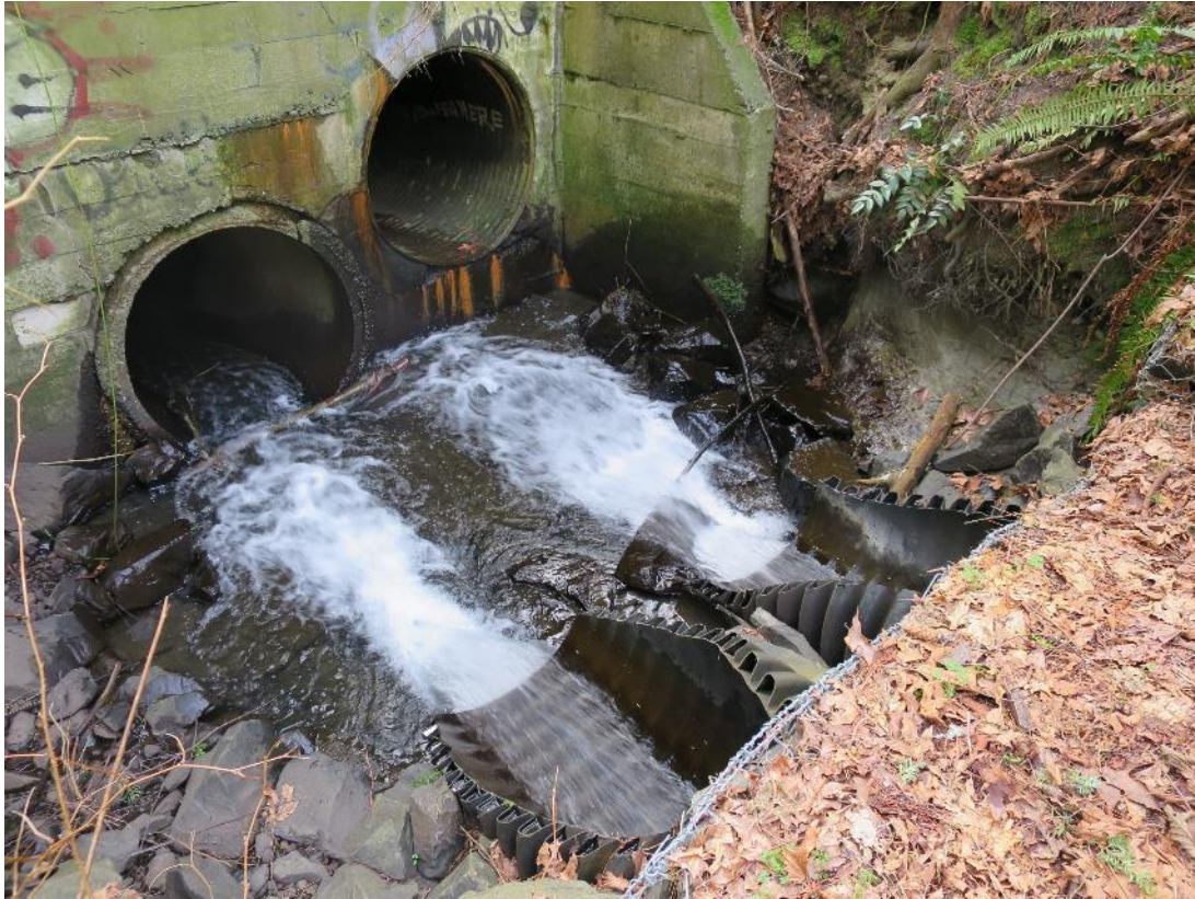
Upstream end of culverts under NW Innis Arden Way
