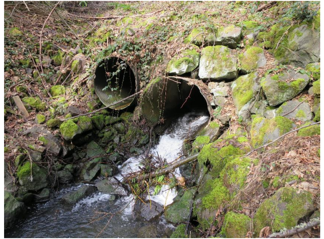
Downstream end of culverts
