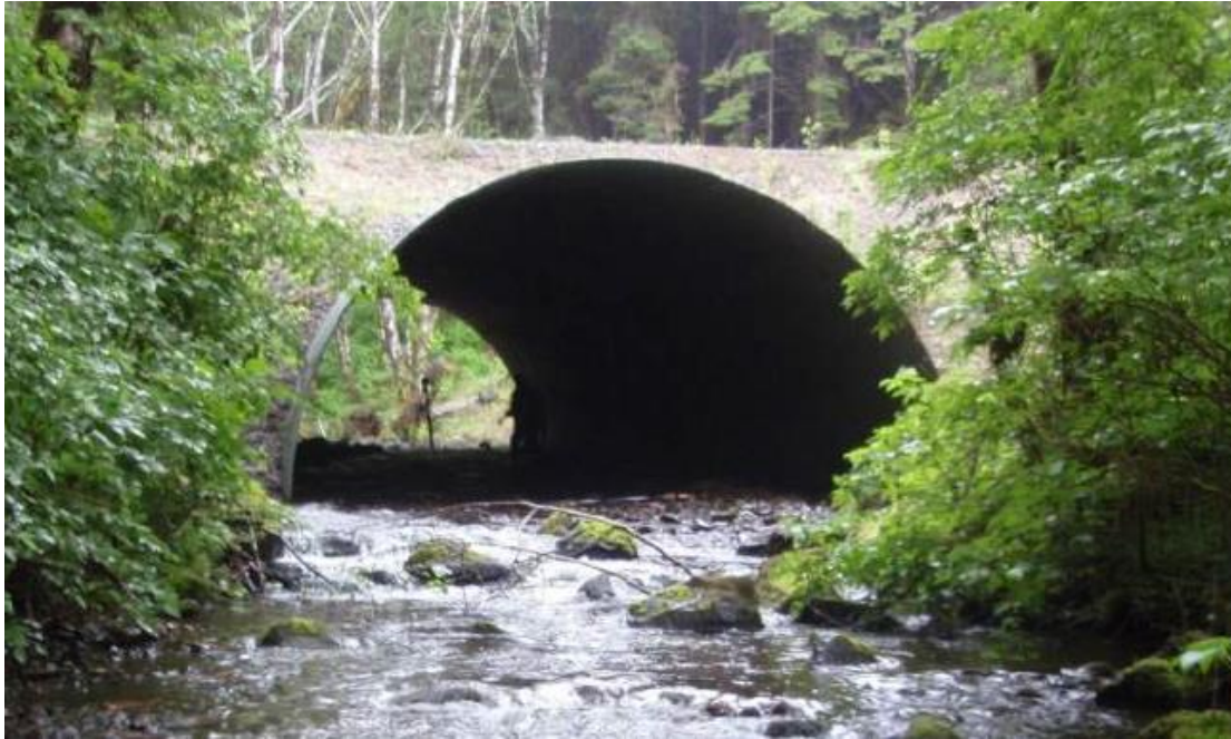
Similar type of culvert as being designed
