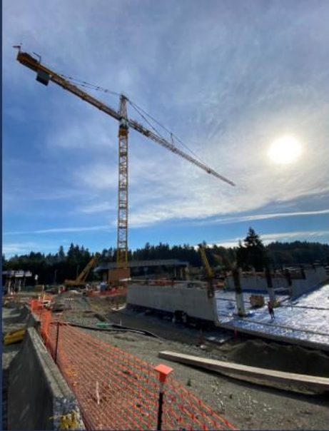
148th Station Garage
