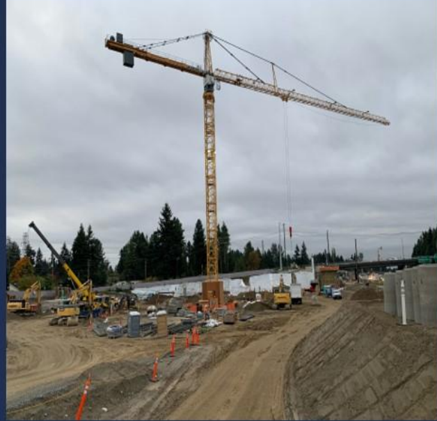
185th Station Garage
