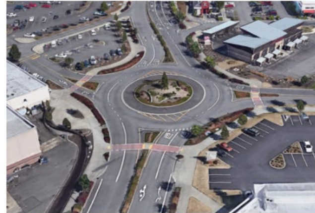
Two-lane roundabout in Covington, WA.
