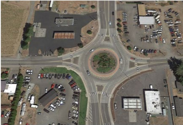
Two-lane roundabout in Lynden, WA.
