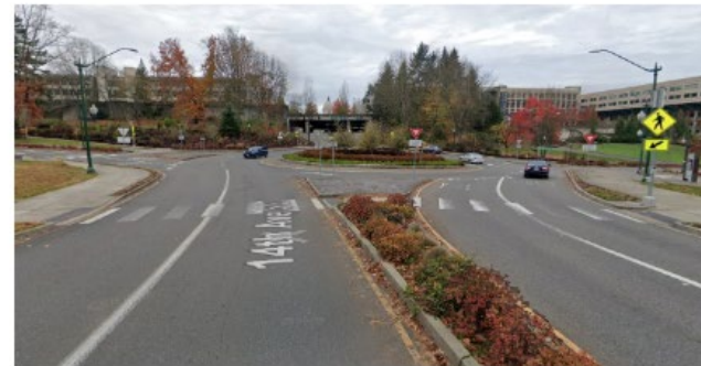
Two-lane roundabout in Olympia, WA looking west.
