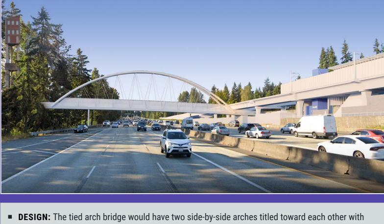
options. ■ SAFETY: The throw barrier could be attached on either side of the cables to prevent things from
