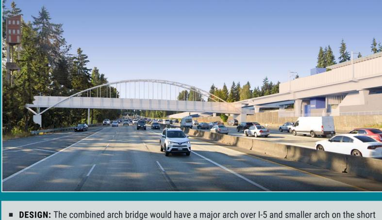
■ SIZE: The arches would have steel support pieces overhead and vertical support pieces that could be cable or steel.
