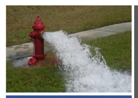
Potable Water Discharges to City Right-of-Way Discharges to the City's stormwater system from potable water sources, including but not limited to water line flushing, hyper chlorinated water line flushing, fire hydrant system flushing, and pipeline hydrostatic test water, are conditionally allowed under the City's municipal stormwater permit. Planned discharges shall meeting the following requirements:
