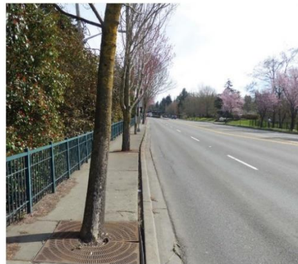
Parts of 175th Street cannot accommodate all users, such as those using strollers and wheelchairs.
