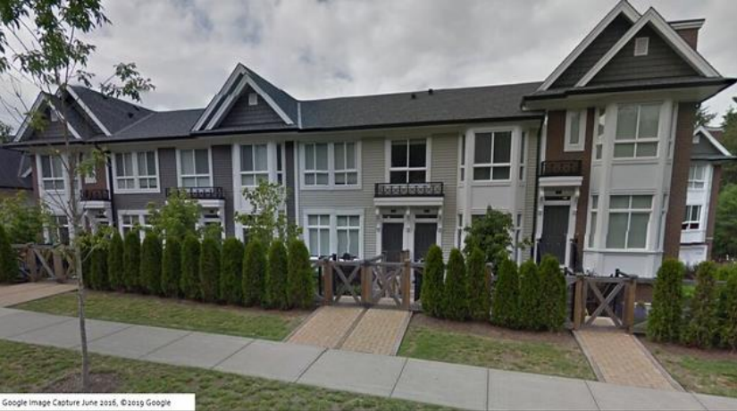
Ranked #1: Front yard landscaping with screening
