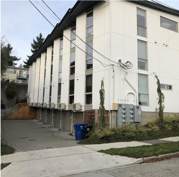
Ranked #2: Trash, recycling and compost is stored in an outdoor enclosure and collected from the driveway
