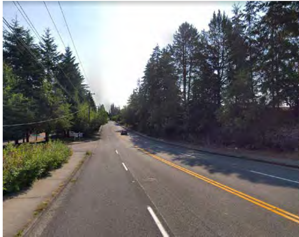
Existing N 160th Street looking East Frontage to be maintained
