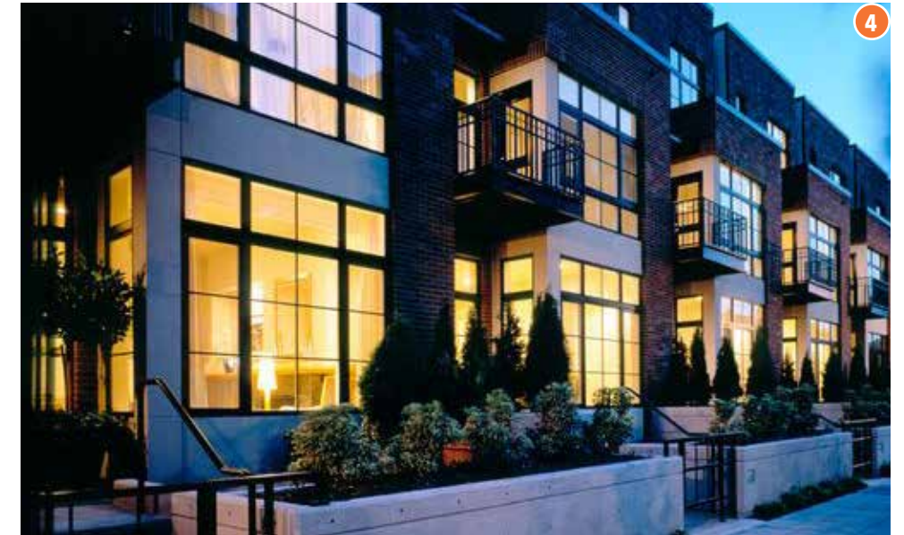
Ground Level Stoops
