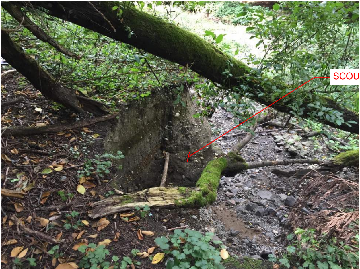
FACING NORTHWEST, FROM TOP OF EXISTING ACCESS RAMP
