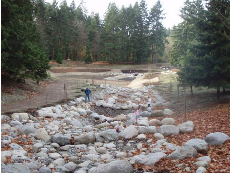
Boeing Creek Park Outfall – 2008, following construction
