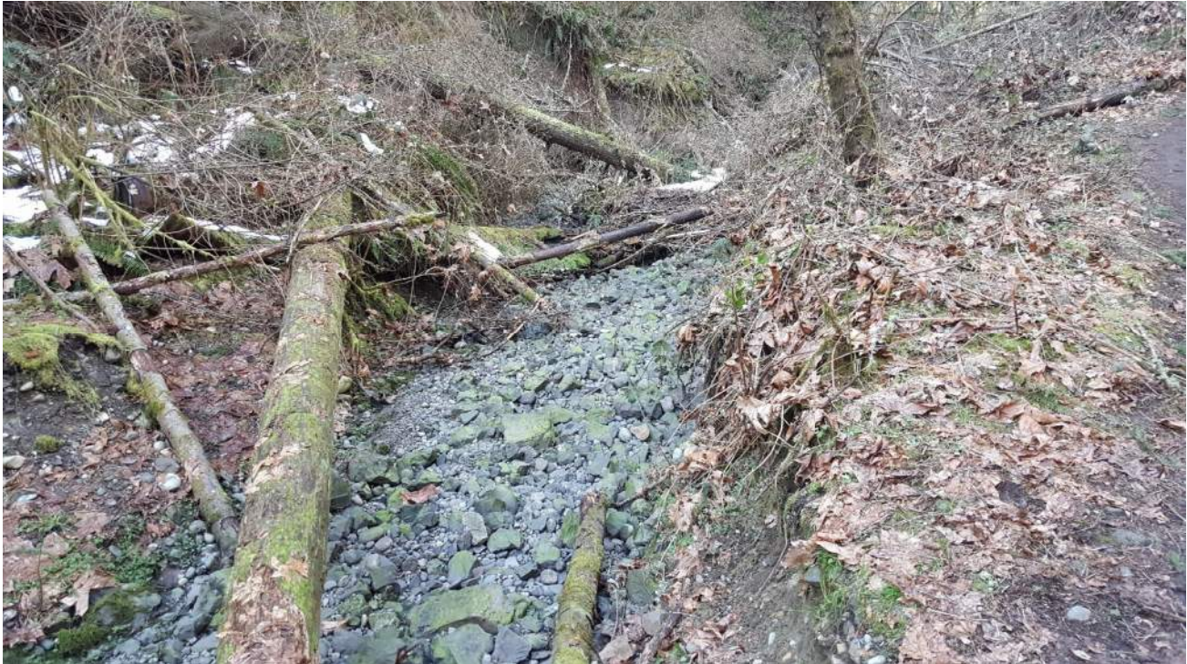
Photo 13. Looking downstream, at the eroded channel, eroded ravine slopes and fallen trees downstream of the M1 Dam.
