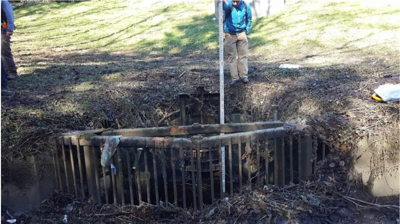
Photo 11. Sluice gate at the outlet pipe of the M1 Dam.
