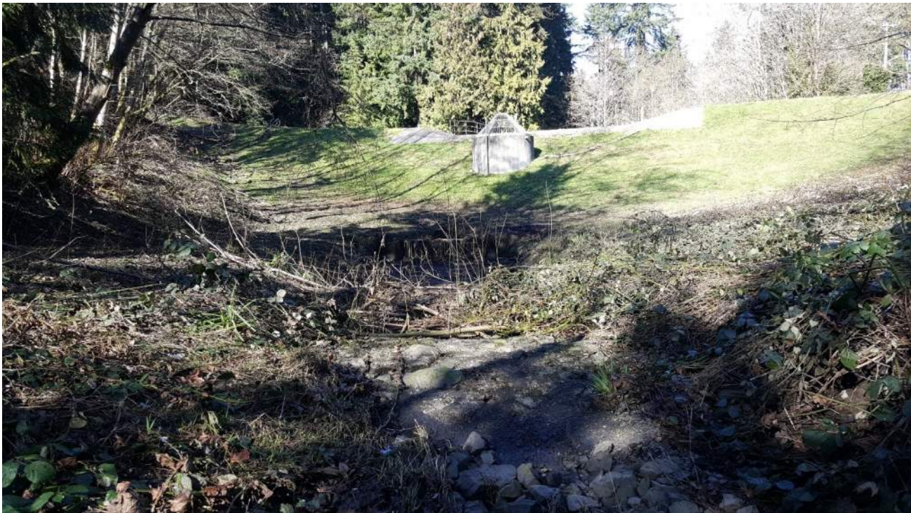
Photo 10. Looking downstream, at the gouted riprap grade control structure, and the M1 dam.
