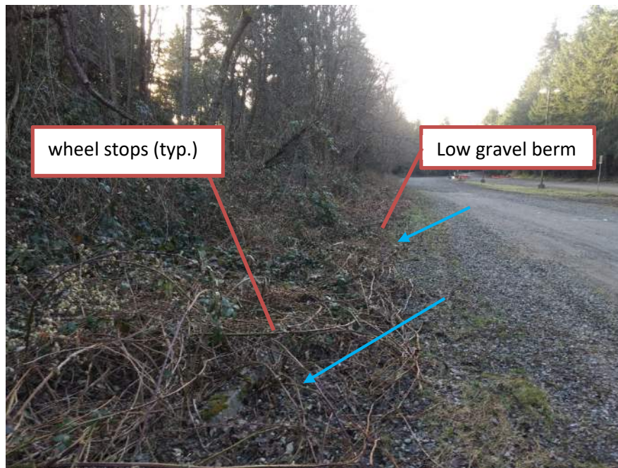
Photo 18: Northeast edge of gravel parking lot (facing southeast)
