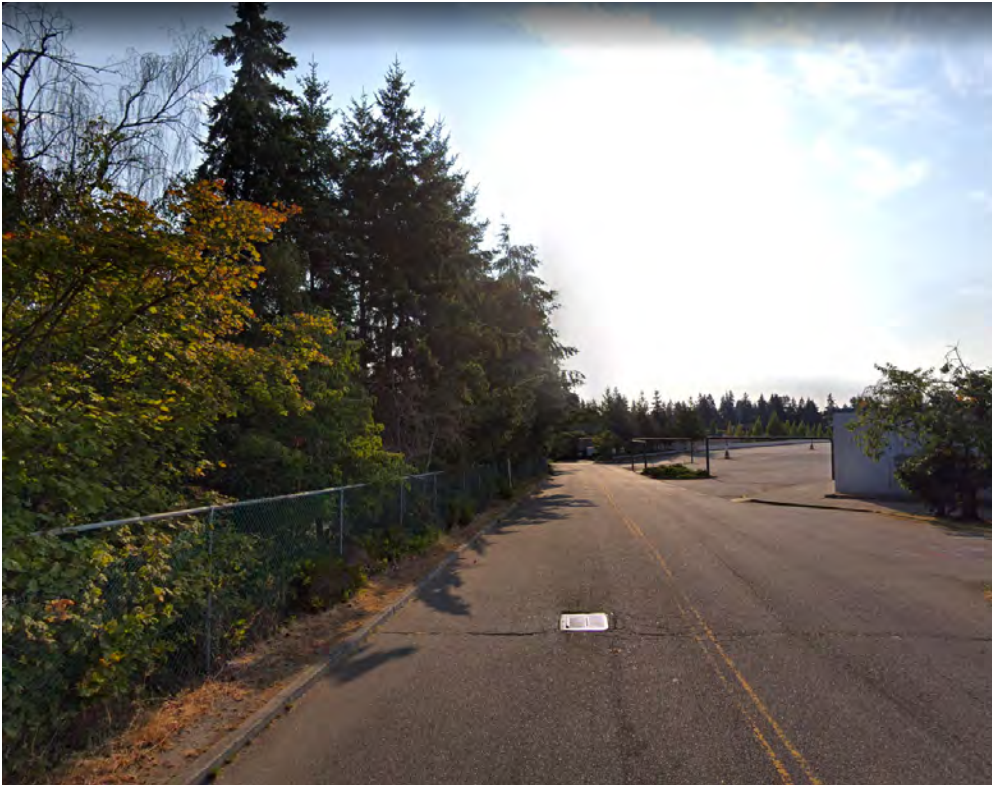
Existing Private Drive along 160th Looking East
