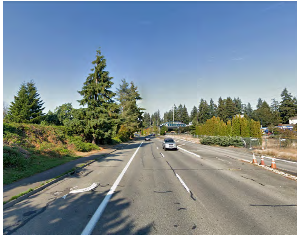
Existing Westminster Way N Looking East
