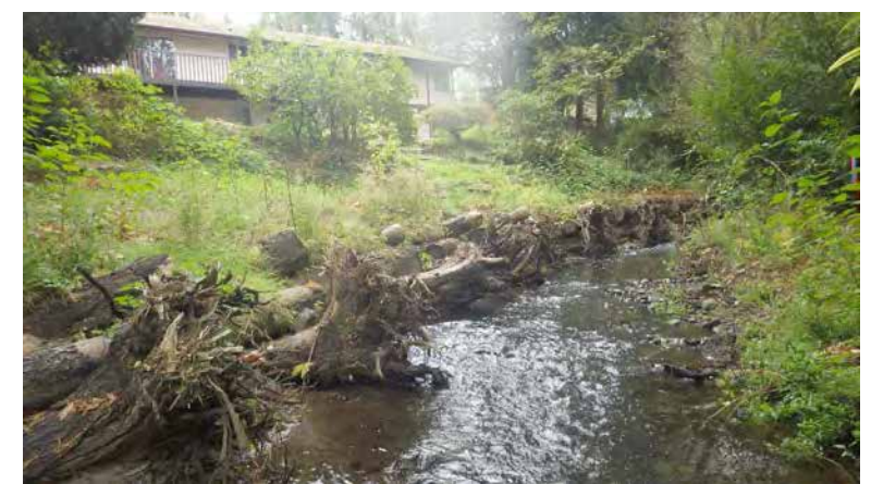
TYPICAL LOG REVETMENT
