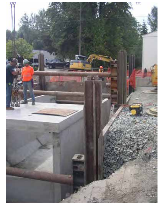
TYPICAL PRECAST BOX CULVERT INSTALLATION
