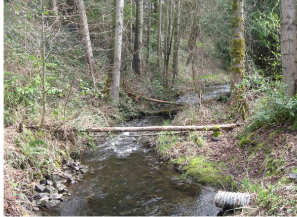
McAleer Creek near the outlet of the culvert under I-5, looking downstream (culvert at right is not the I-5 culvert)
