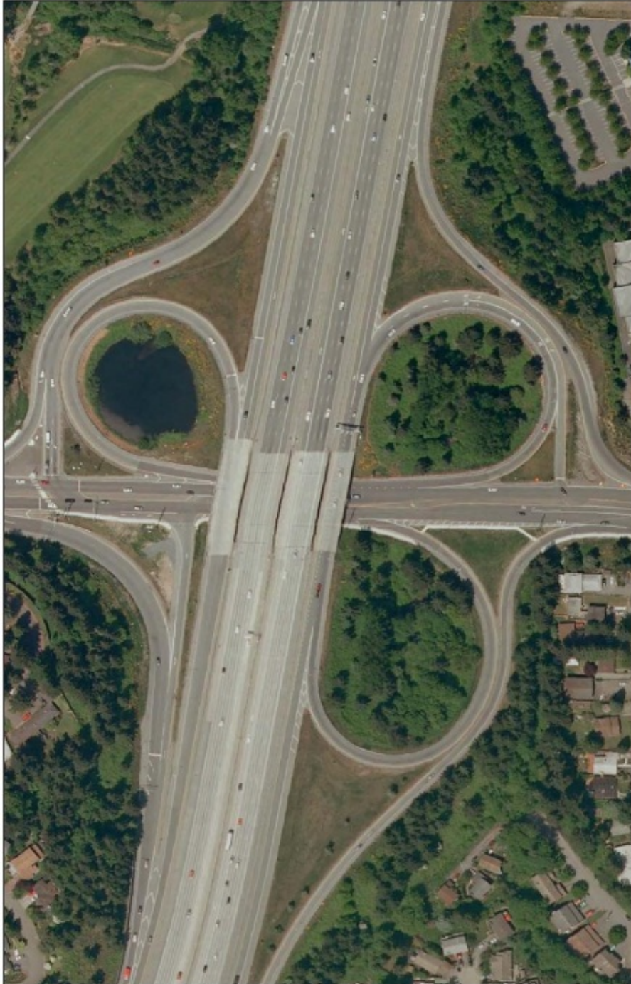
Figure 9. SR 104 (NE 205th Street) Interchange
