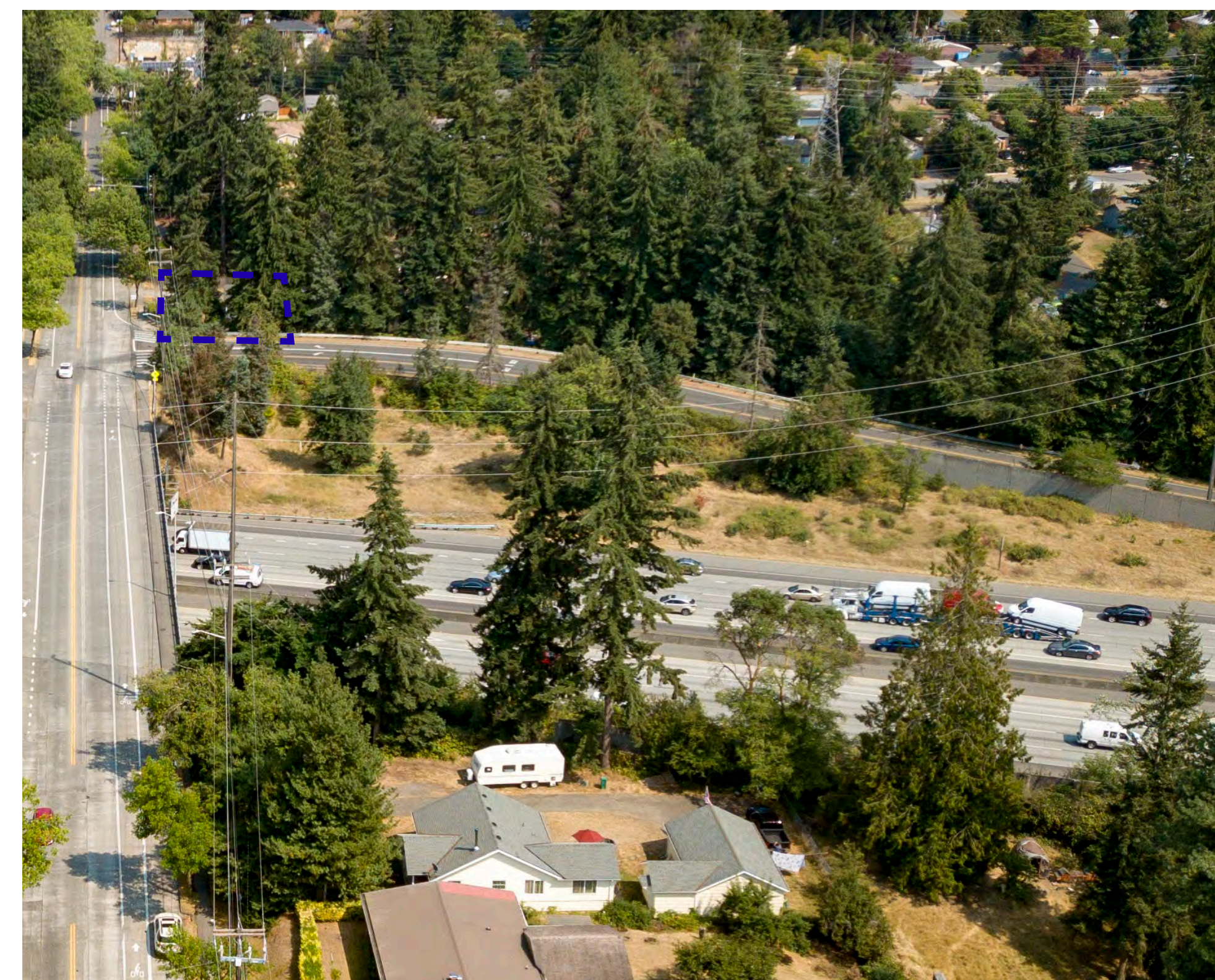
AERIAL VIEW OF SITE
