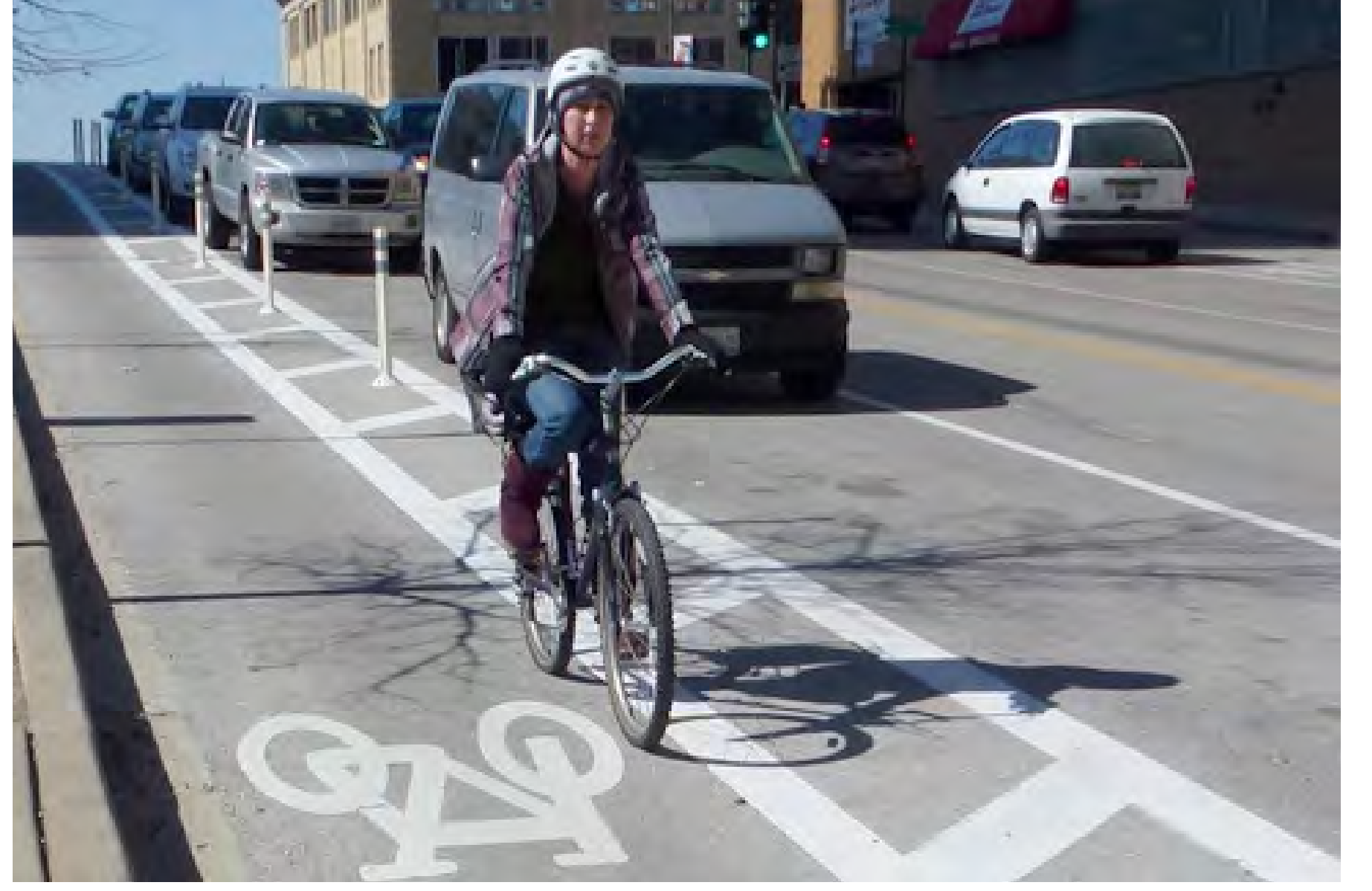
PROTECTED BIKE LANE WITH BOLLARDS IN BUFFER
