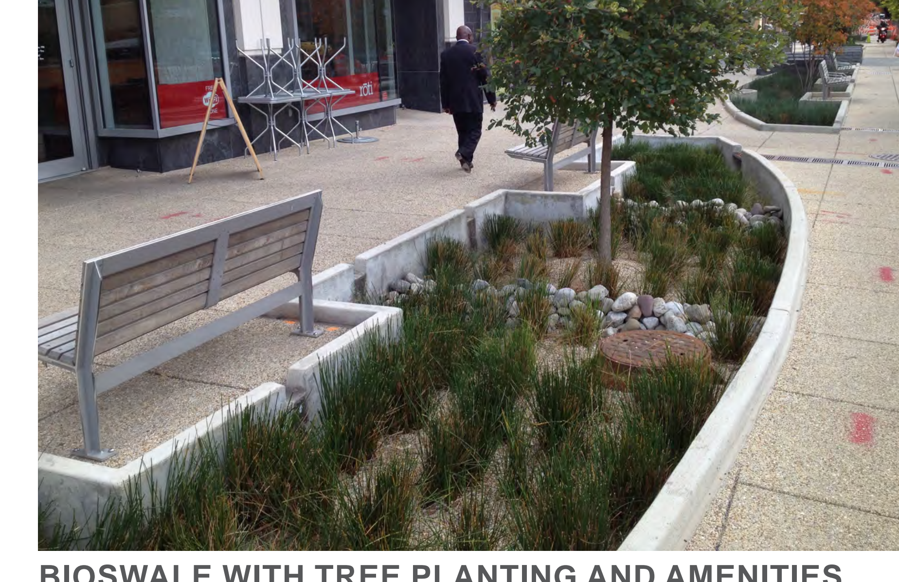
BIOSWALE WITH TREE PLANTING AND AMENITIES
