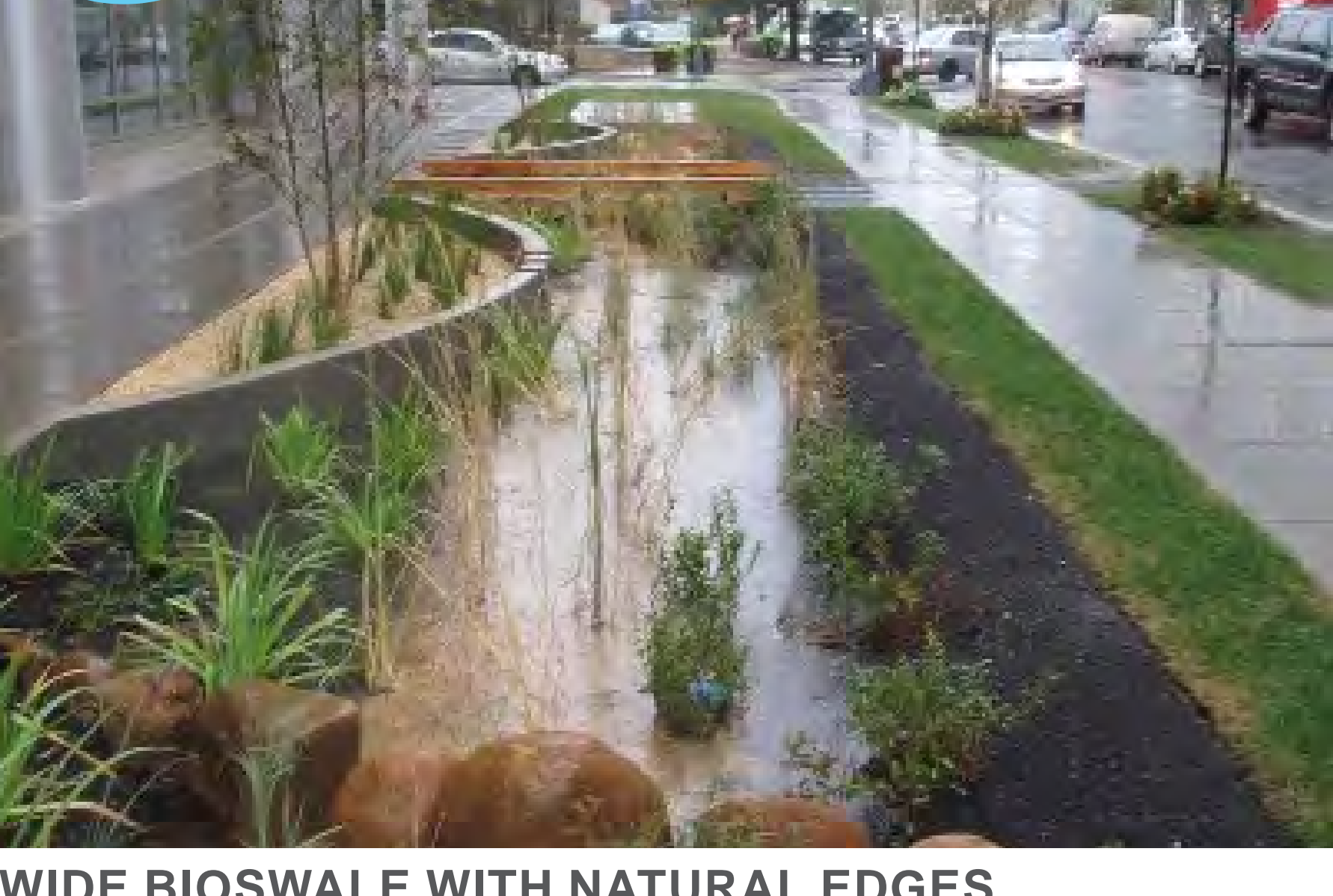
WIDE BIOSWALE WITH NATURAL EDGES
