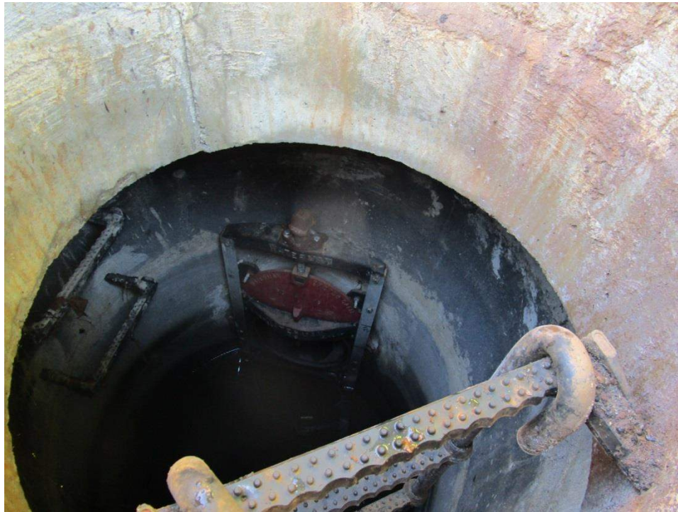
Figure 6: CB-12420 and Partially Closed Valve
