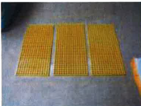
(1) Bottom Grates found in chamber
