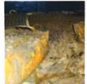
Figure 2. Perlite filter media needs replacement.
