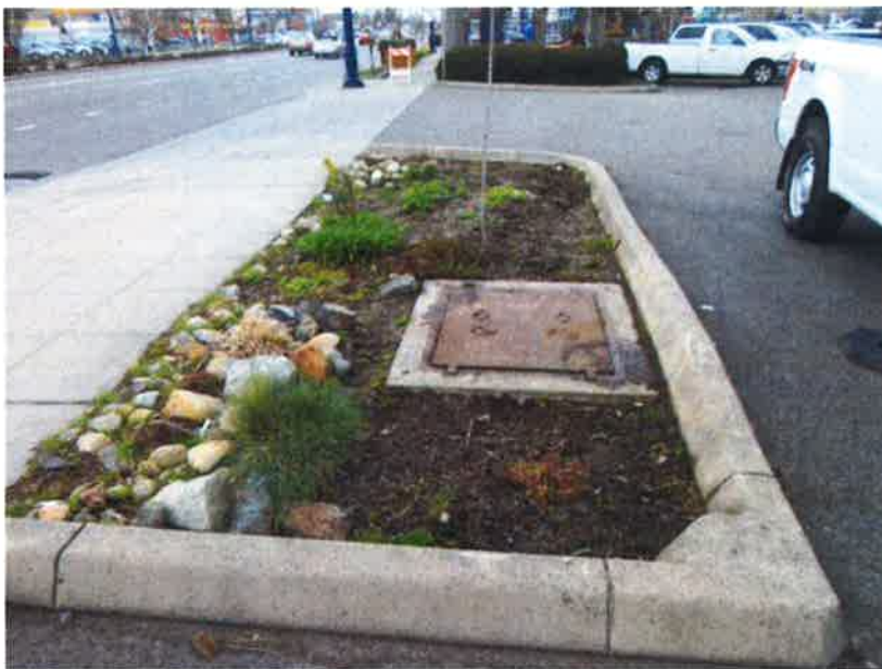
Figure 4-16. Oil/water separator
