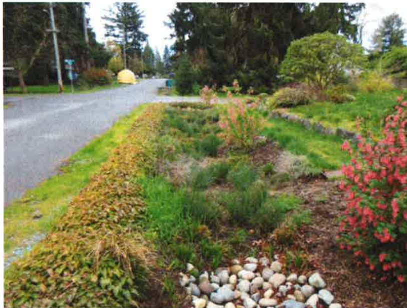
Figure 4-1. Bioretention facility
