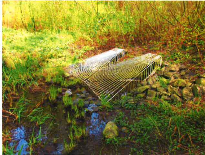
Figure 4-20. Pipe inlet structure
