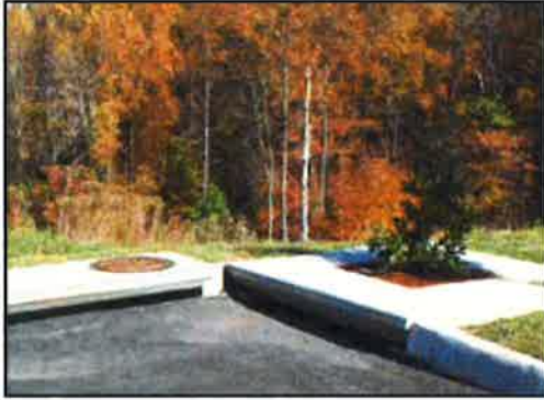
1. Inspection of Filterra and surrounding area
