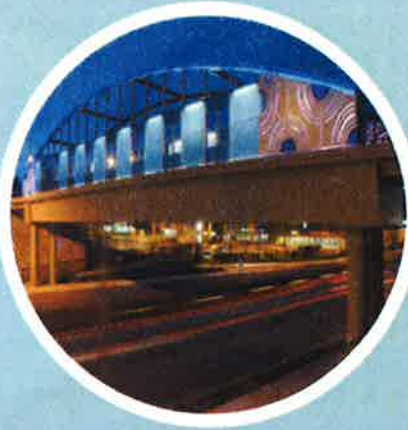
Aurora Avenue N Bridge
