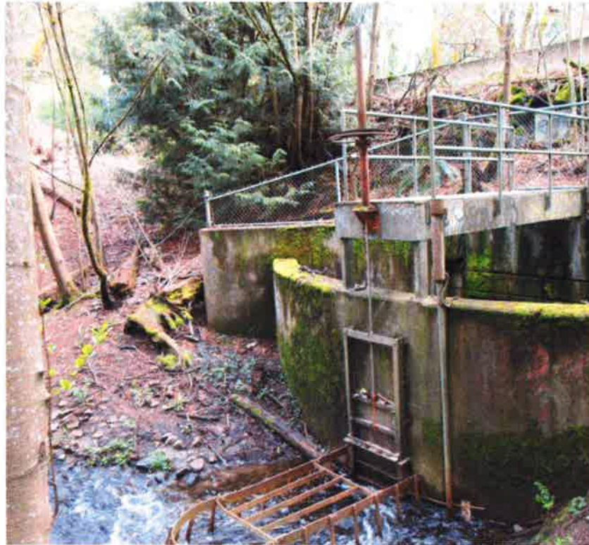
Figure 4-11. Gate valve
