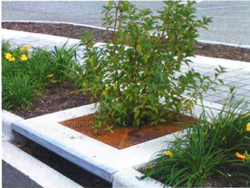
Figure 4-10. Filterra
