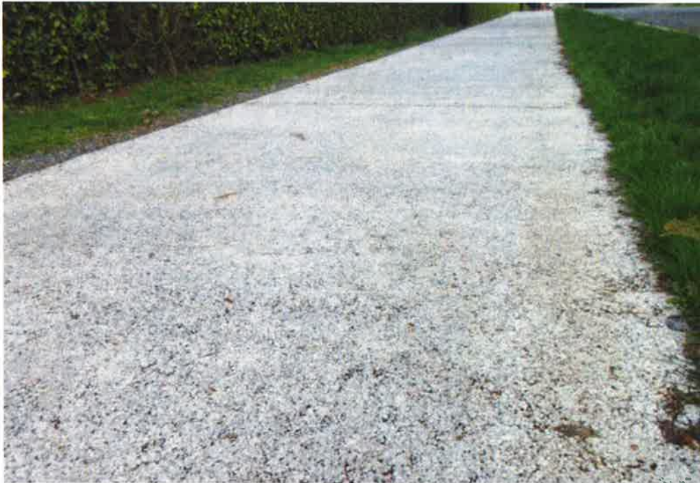
Figure 4-18. Permeable pavement
