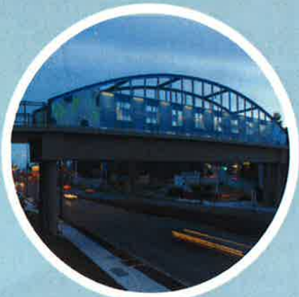
Aurora Avenue N Bridge
