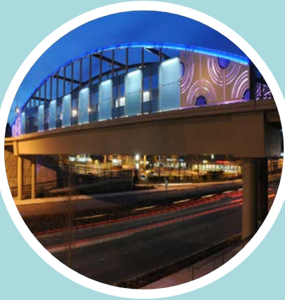
Aurora Avenue N Bridge
