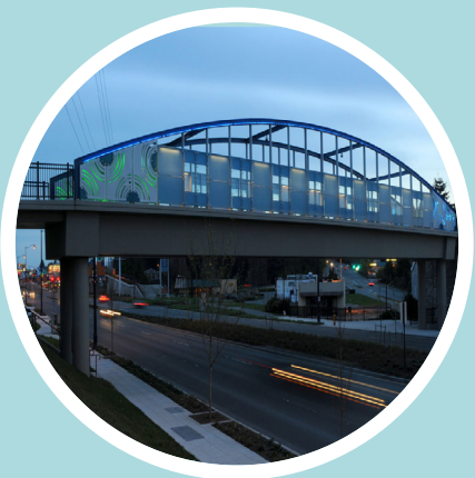
Aurora Avenue N Bridge
