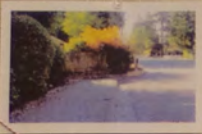
Sidewalk abruptly ends
