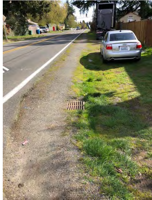
194th and 1st NE looking south
