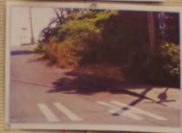
Missing sidewalk connection to Interurban Trail
