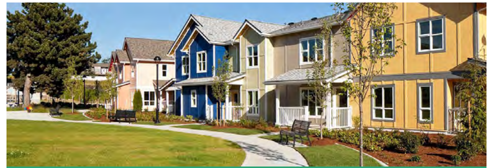
Affordable Housing in Bend, Oregon
