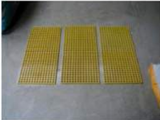
(1) Bottom Grates found in chamber
