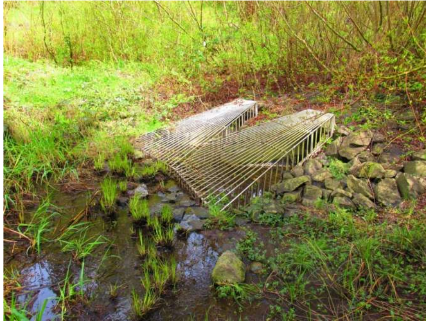
Figure 4-20. Pipe inlet structure
