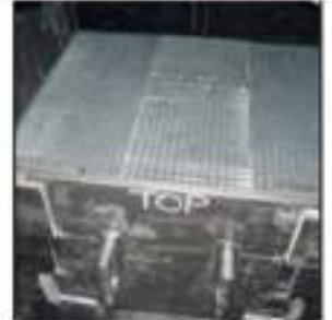
Figure 1. Removable bulkhead door across from ingress/egress ladder at rear of filtration chamber.
