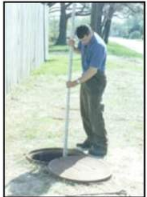
Sediment inspection using a stadia rod in a single pretreatment chamber.
