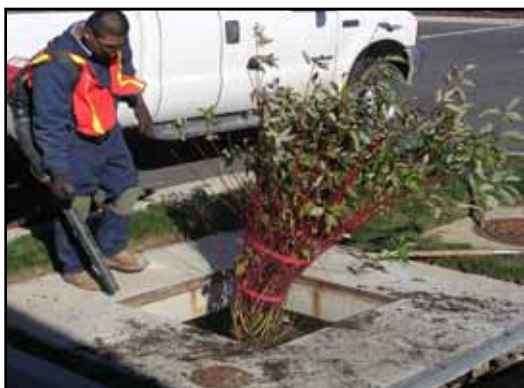
5. Clean area around Filterra
