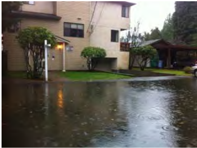
Photo 1 – November 19, 2012 Rain Event Ponding along 148th*
