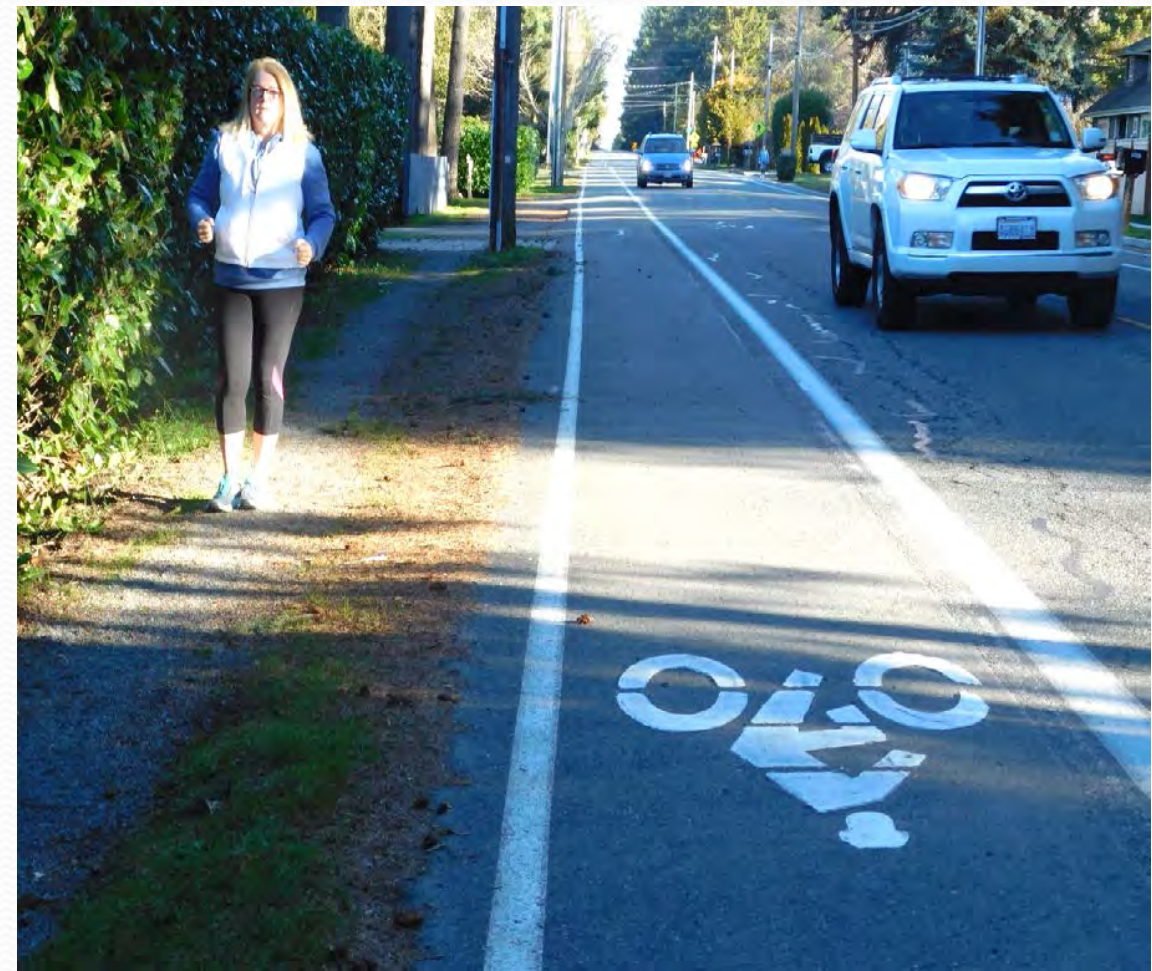
Gravel Path Provides More Separation From Traffic
