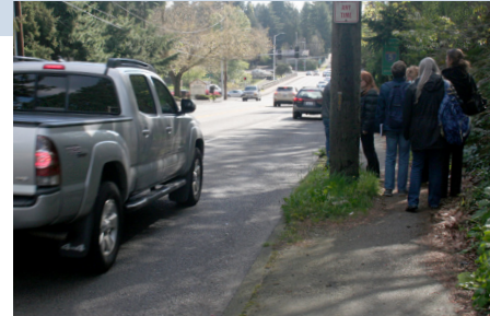
Poorly placed utility poles reduce sidewalk width
