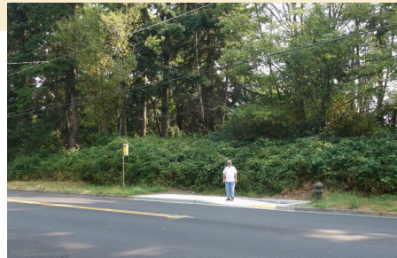
Missing sidewalk and crosswalk connections to and from bus stop
