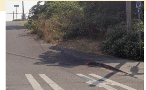
Missing sidewalk connections to the Interurban Trail
