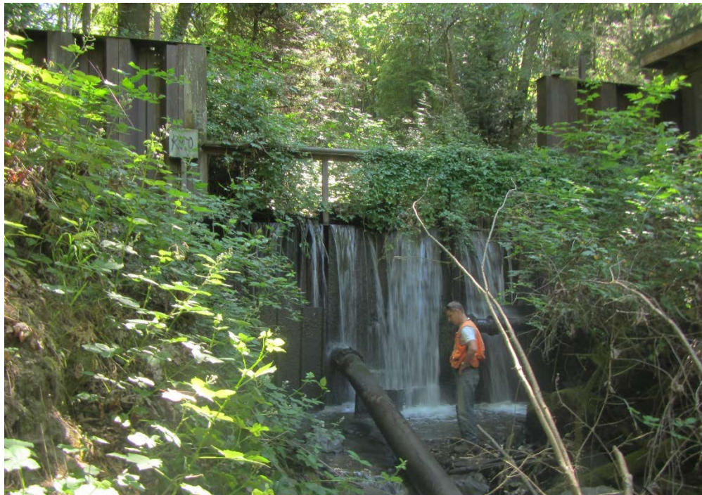
Figure 3. Looking Upstream at Seattle Golf Club Diversion Dam.
