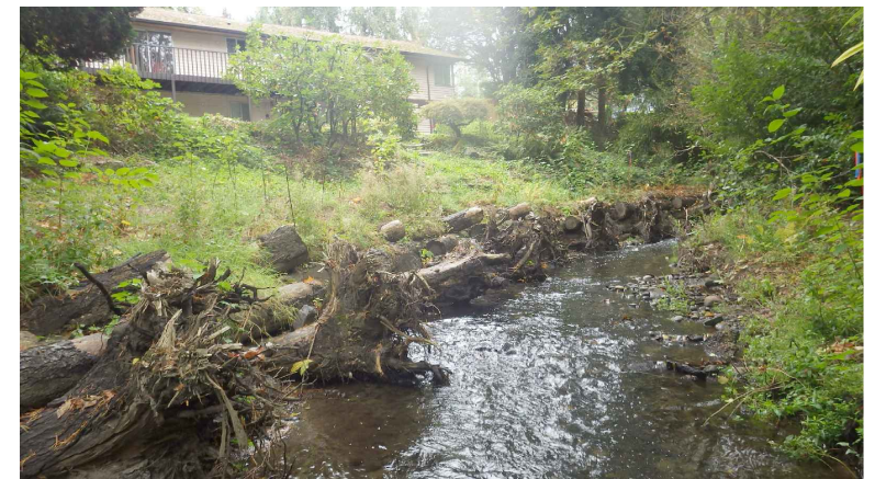
TYPICAL LOG REVETMENT
