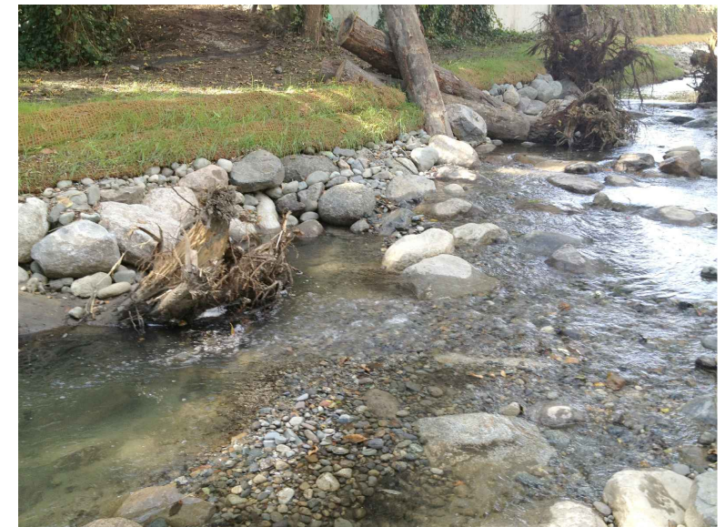
TYPICAL ROCK/COIR WRAP EMBANKMENT
