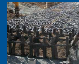
▲ Installation of root box system under the sidewalk
