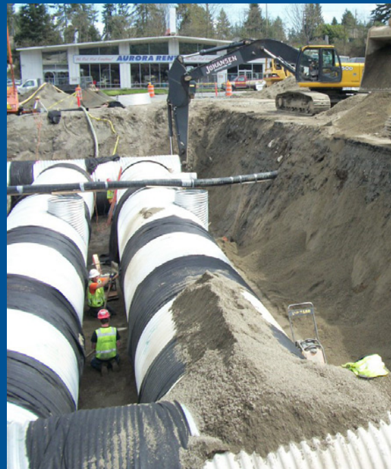
▲ Construction of the pipe farm under this plaza
