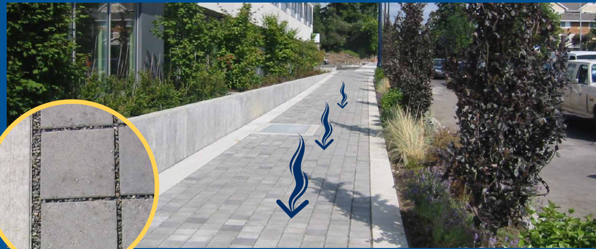
▲ Permeable sidewalk pavers (root box system underground) and a planting bed line the south side of Shoreline City Hall.
