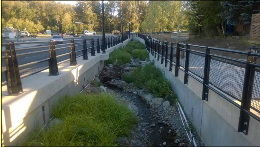
Photo ES-1. Example of 3-Sided Open Channel with Concrete Walls
