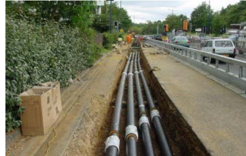
DISTRIBUTION PIPING 4 pipe system (heating & cooling)
