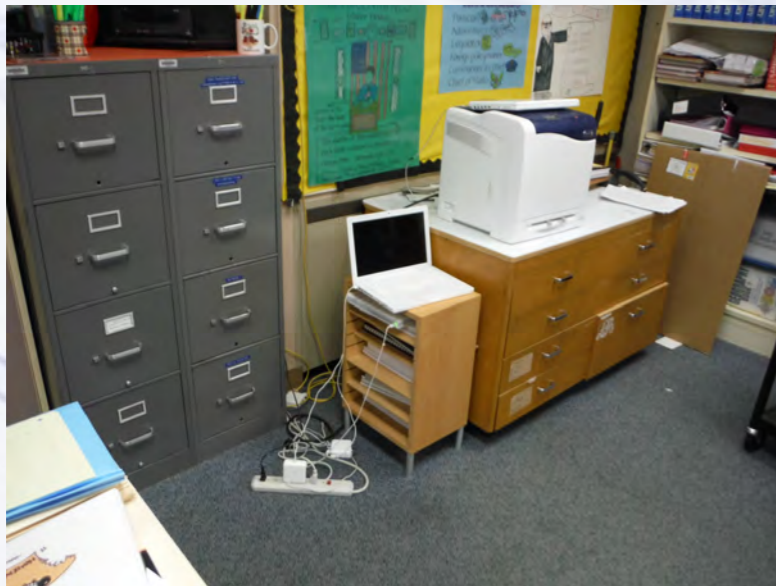
Electrical – not enough outlets
