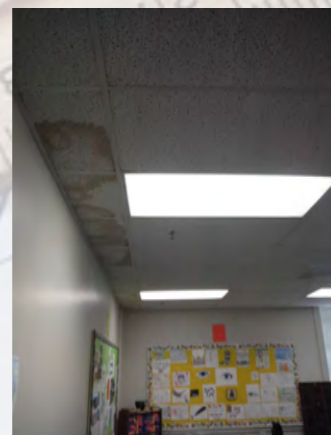
Roof leaks
