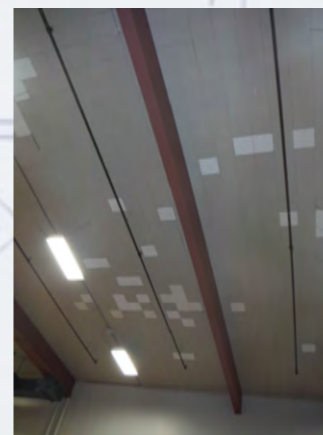
Roof leaks
