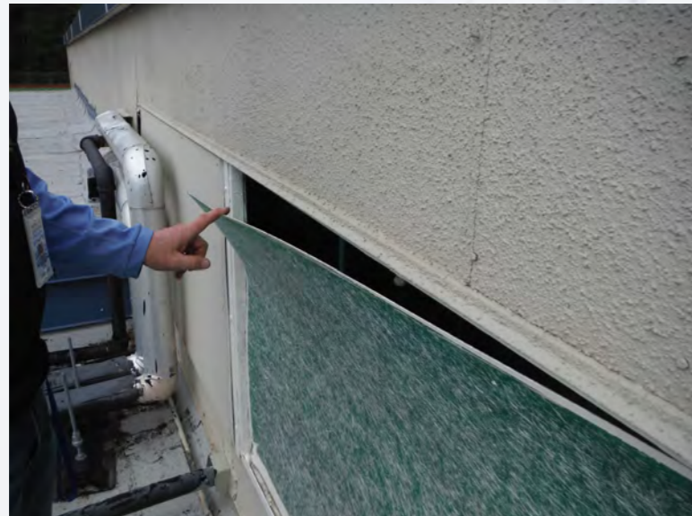
Art Building – window panels
