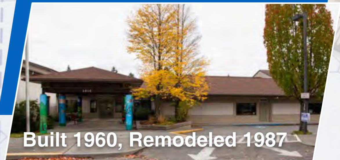
Rebuild Parkwood Elementary School
