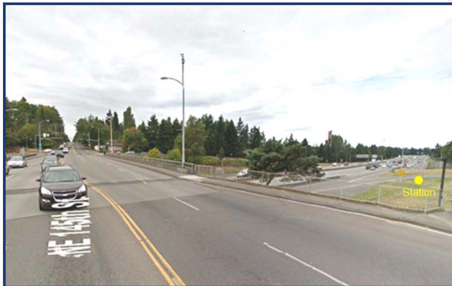
Figure 4-12: Looking Northwest from 145th Street / Link Light Rail Station
