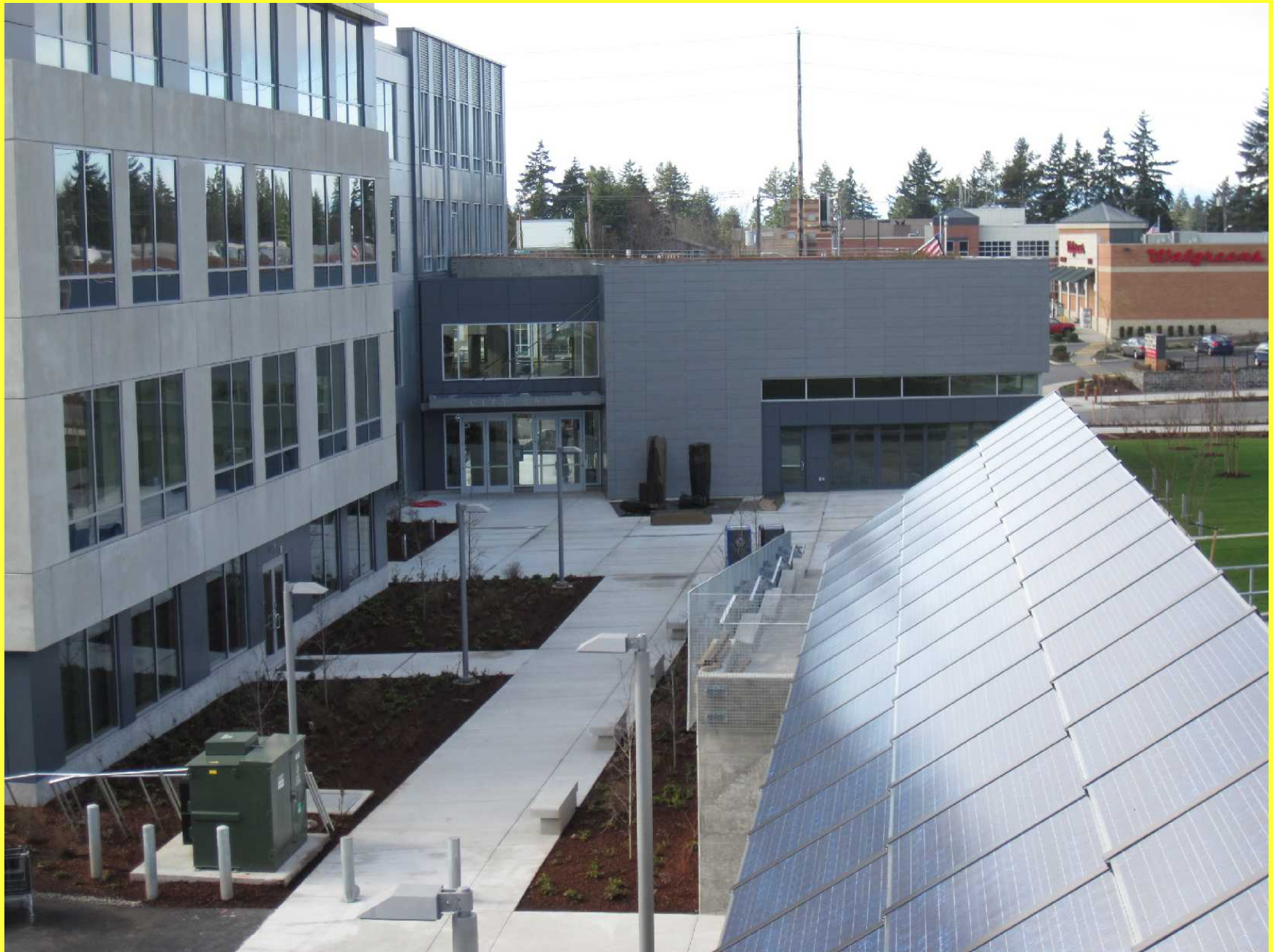
Shoreline City Hall (Looking West)
