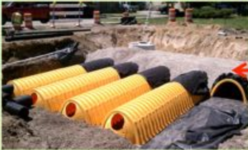
Stormwater Vault
